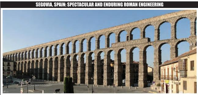
The Roman aqueduct in Segovia, Spain, stands as one of the most well-preserved and astounding engineering feats of the Roman Empire. Constructed around the 1st century AD, it soars to a height of 93.5 feet (28.5 meters). Remarkably, no mortar was used in its assembly. The granite blocks were meticulously cut and expertly balanced, enabling the aqueduct's continuous operation in delivering water to the city until the 19th century.
