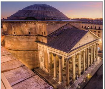
Rome's Pantheon, as rebuilt by the emperor Hadrian in 120 AD. The massive structure is still the world's largest reinforced concrete dome. The interior, left, contains an occulus in its center, which relieves the pressure on the rook and provides the sole source of internal light. Each year on April 21st, traditionally considered the foundation date of Rome, sunlight strikes the doorway at precisely midday, a deliberate structural design element.
