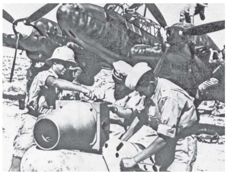
Detaching the film canister from the *Rb* 50/30 camera of a *Bf* 110C-5 reconnaissance aircraft.
