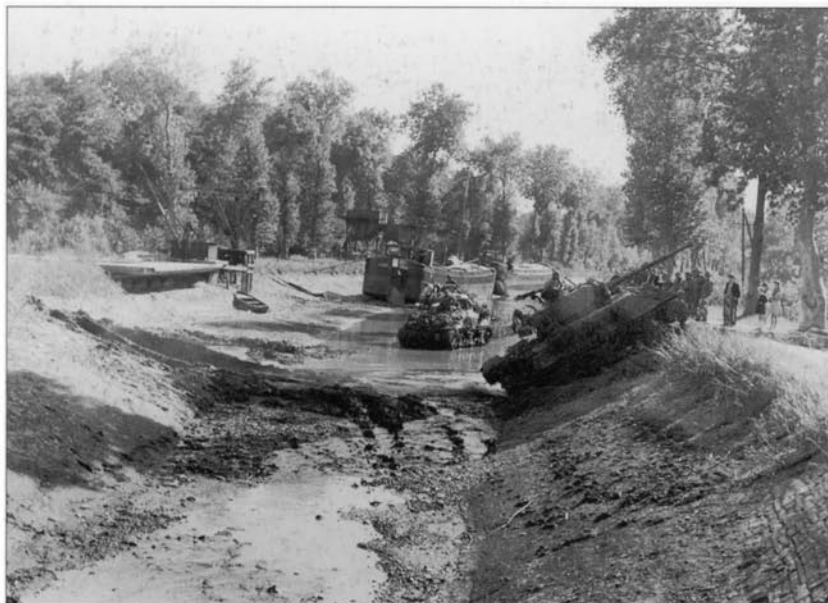
The 8th Tank Bn. crossing of the Bayon Canal was made possible by the low water level in several sections. This is evident here as several of the barges are left high and dry in the mud. The M4 exiting the canal is one of the newer M4 medium tanks armed with the long 76mm gun. These were not in widespread service in the 4th Armd. Div. at the time, since Patton did not feel that they were necessary. (US Army)
