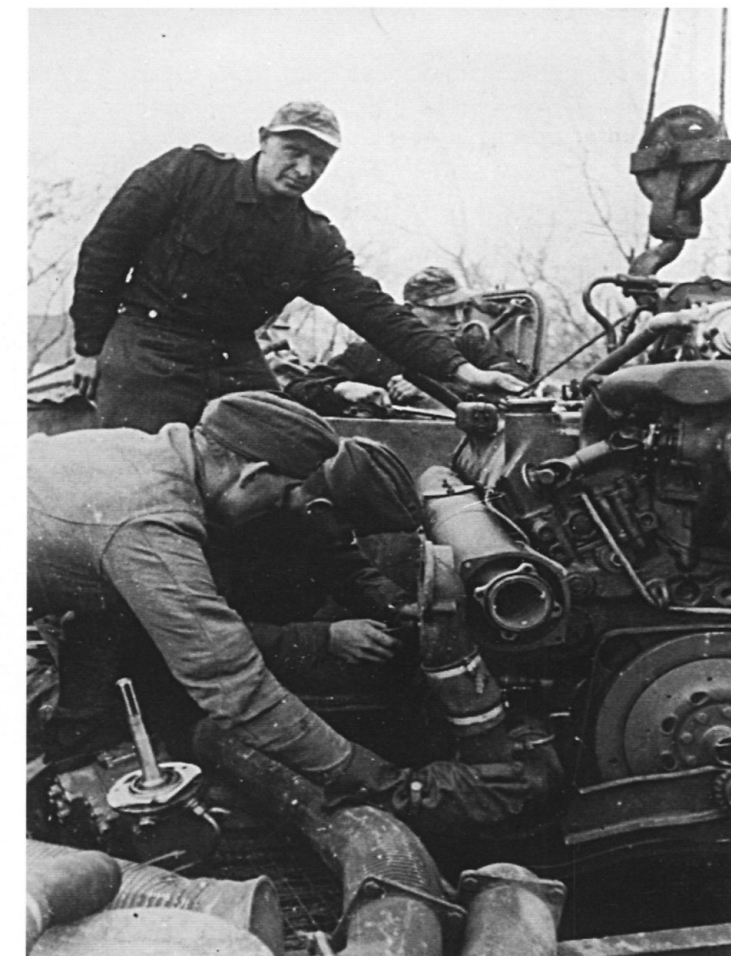
SS mechanics belonging to a field maintenance company replace the Maybach HL230 P45 V12 engine of a Tiger I during the Normandy campaign. The independent Tiger battalions owed much of their success to their well-equipped maintenance companies, which kept the vehicles in fighting condition.
