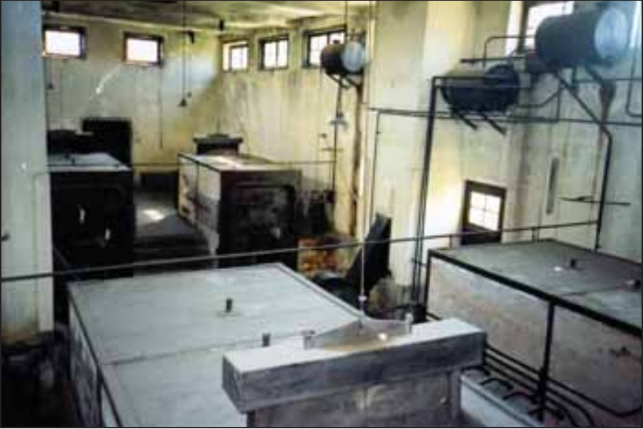
Photograph 345: The four furnaces viewed from above. On the right-hand wall, top, are the naphtha tanks.
