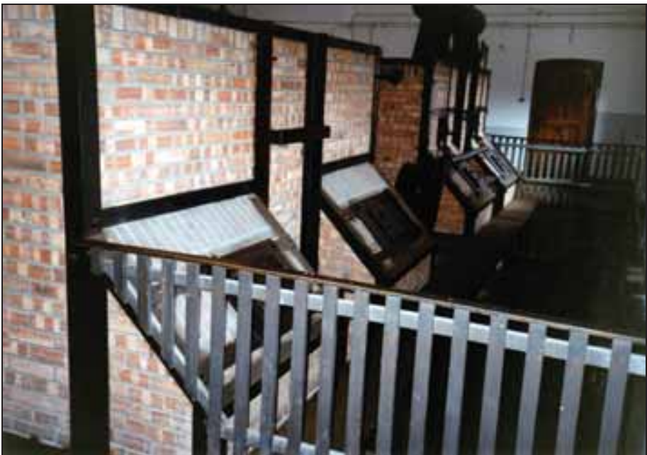
Photograph 205: Rear view of the two TOPF triple-muffle cremation furnaces.
