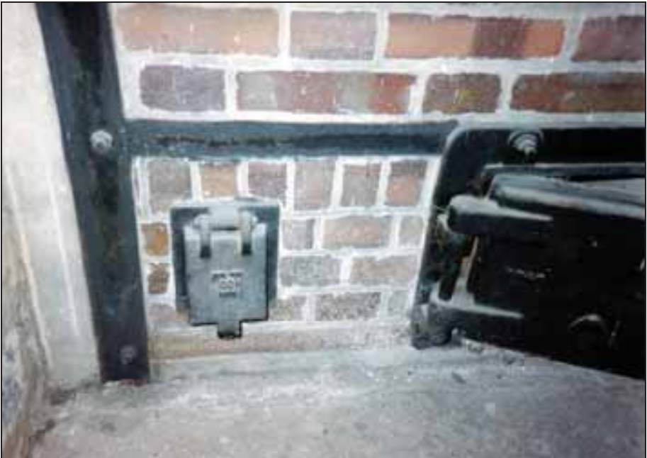
Photograph 81: as above; the left-hand combustion-air-intake door.
