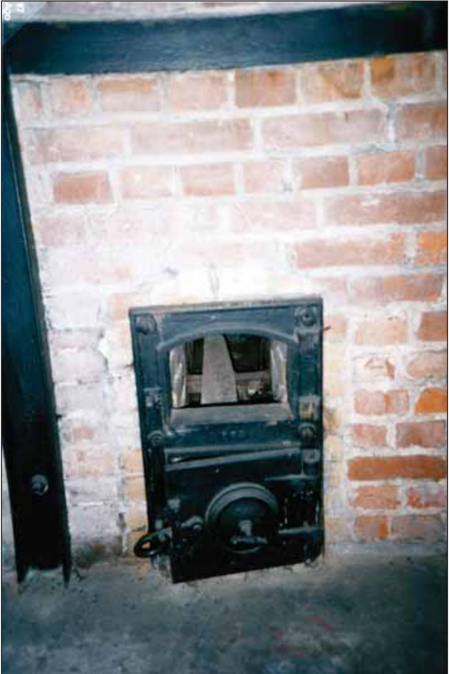
Photograph 280: Left-hand furnace; doors of the auxiliary gasifier.
