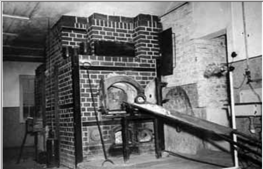
Photograph 336: KORI coke-fired cremation furnace at the Ebensee Camp. Source: www.profit-over-life.org/teachers_guide/austria/mauthausen_kz/mauthausen-ebensee_crematorium.html
