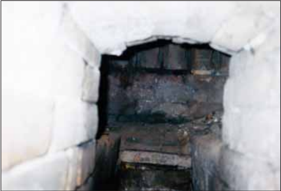
Photograph 283: Right-hand furnace, inside of the auxiliary gasifier with the muffle's ash chamber wall in the background and the muffle grate above.
