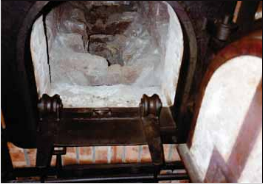
Photograph 179: as above, movable roller device put into place for operation.
