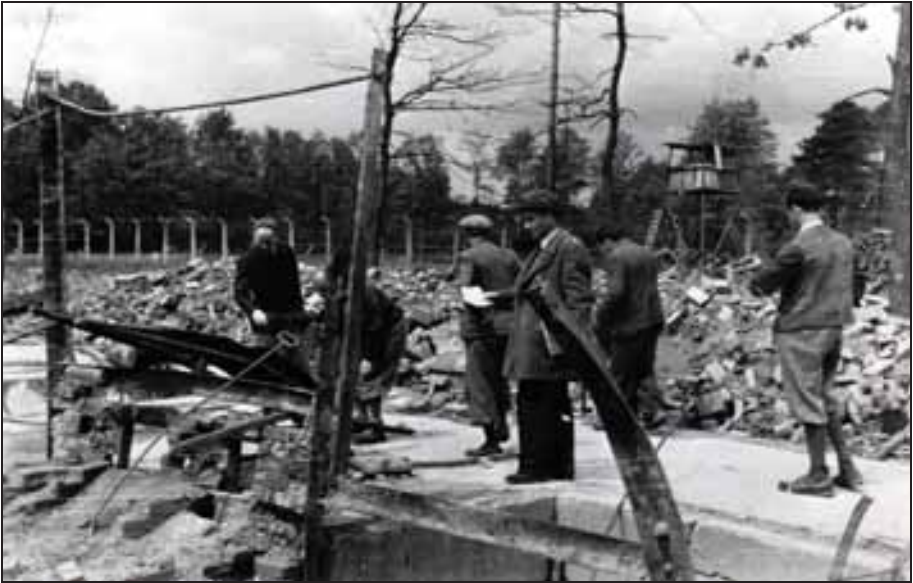
Photograph 225: as above; APMO, negative no. 21334/81.
