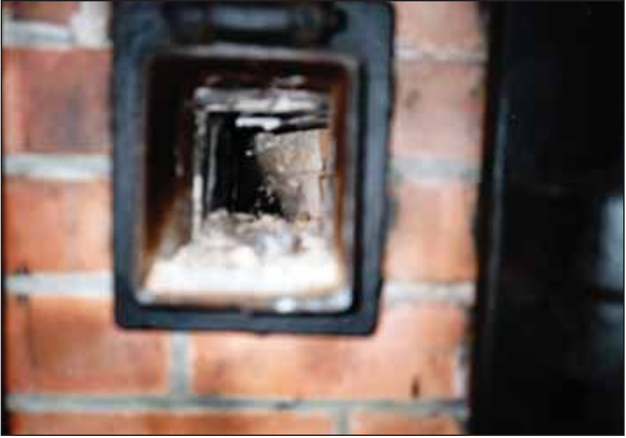
Photograph 151: as above, the muffle's combustion-air-supply channel.
