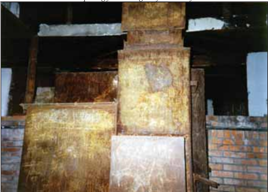
Photograph 48: Central part of the chimney.
