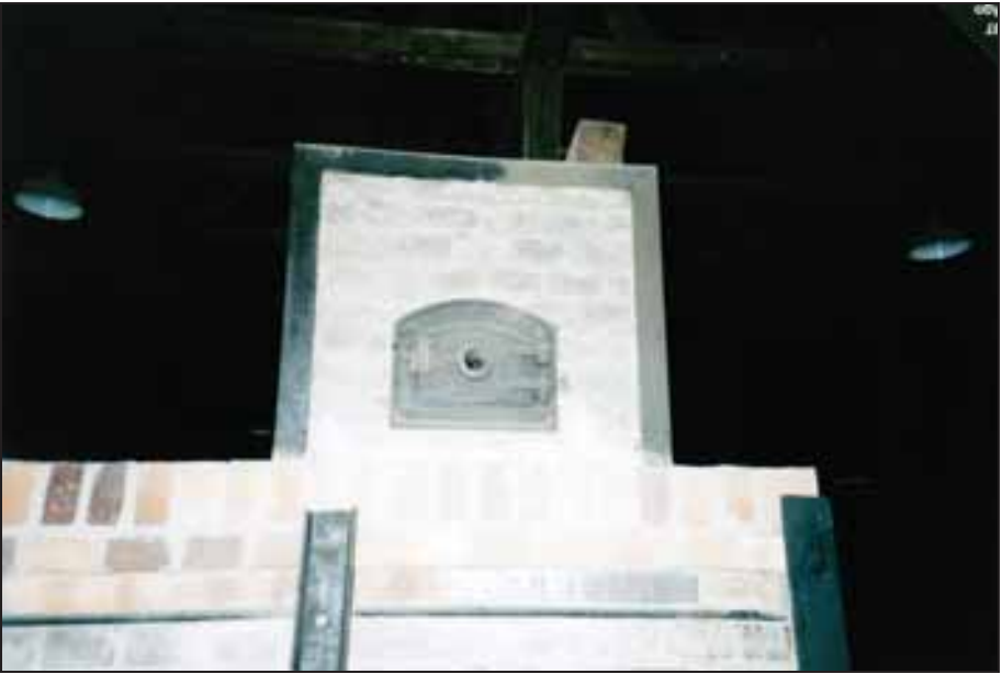
Photograph 310: as above, smoke duct with inspection door.
