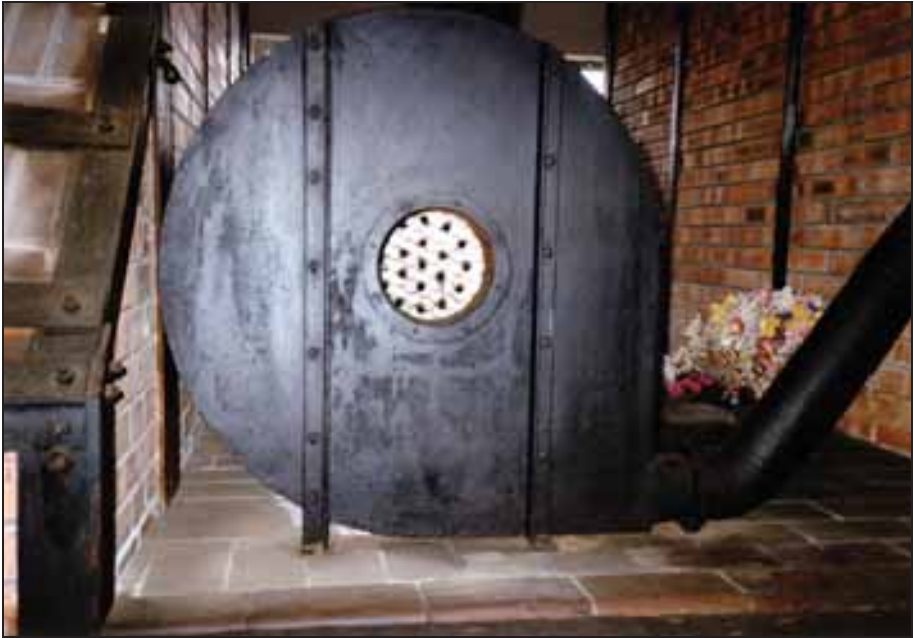
Photograph 195: Combustion-air blower for the oil burner of the furnace heated with either naphtha or coke. Rear view.
