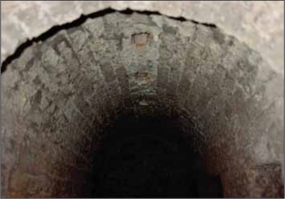
Photograph 143: as above, vaulted muffle ceiling with square openings for combustion-air supply.
