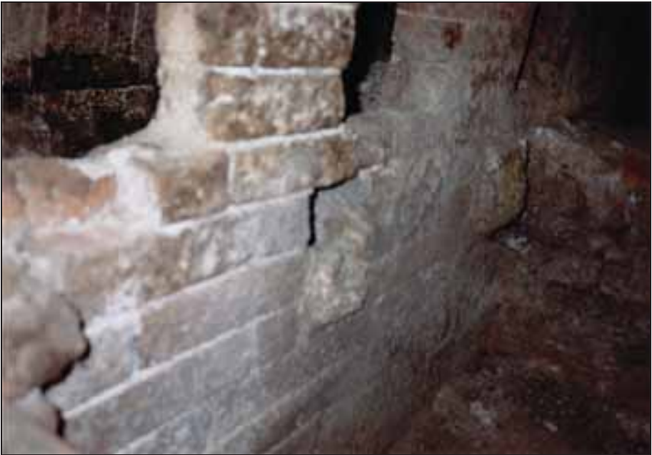
Photograph 23: Right-hand muffle: detail of the partition wall with inter-muffle openings.
