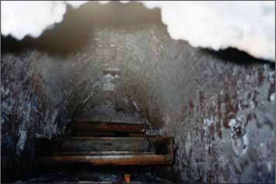
Photograph 352: as above; the muffle's inside seen from its rear service door. In the foreground the front part of the corpse-introduction cart.
