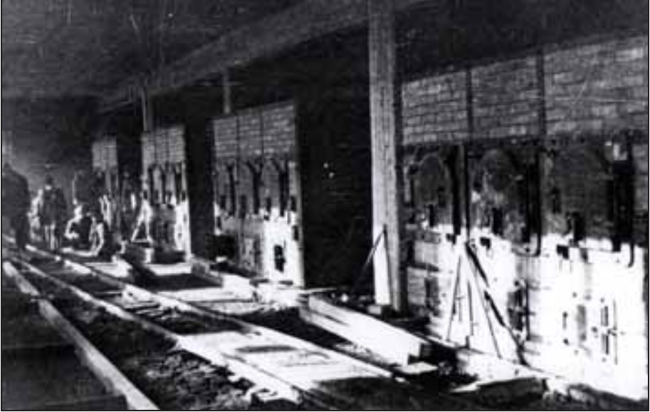
Photograph 111: SS photo of the TOPF coke-fired triple-muffle furnaces at Crematorium II at Birkenau. APMO, microfilm no. 287.
