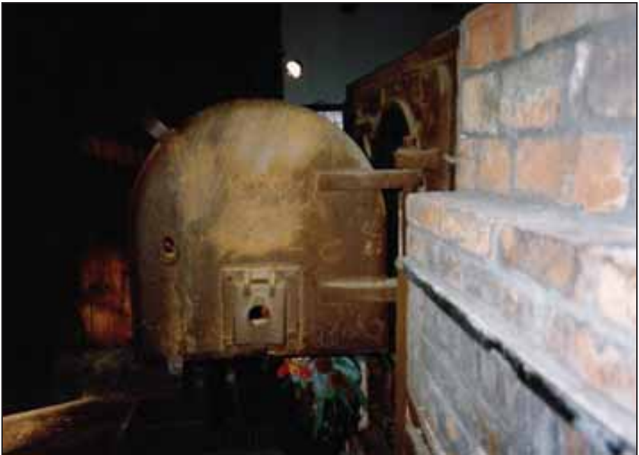
Photograph 44: Outside of left-hand muffle door.
