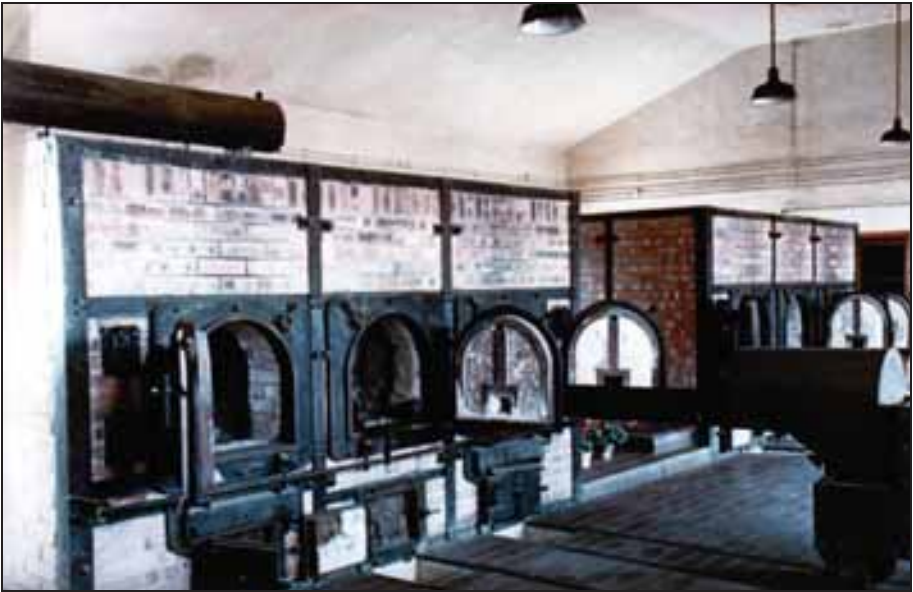
Photograph 116: TOPF triple-muffle cremation furnace in the Crematorium at Buchenwald Concentration Camp.
