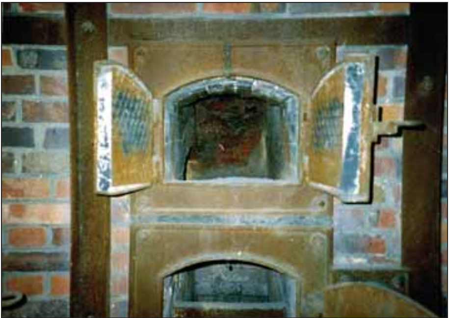
Photograph 261: Coke-loading door of the main gasifier.
