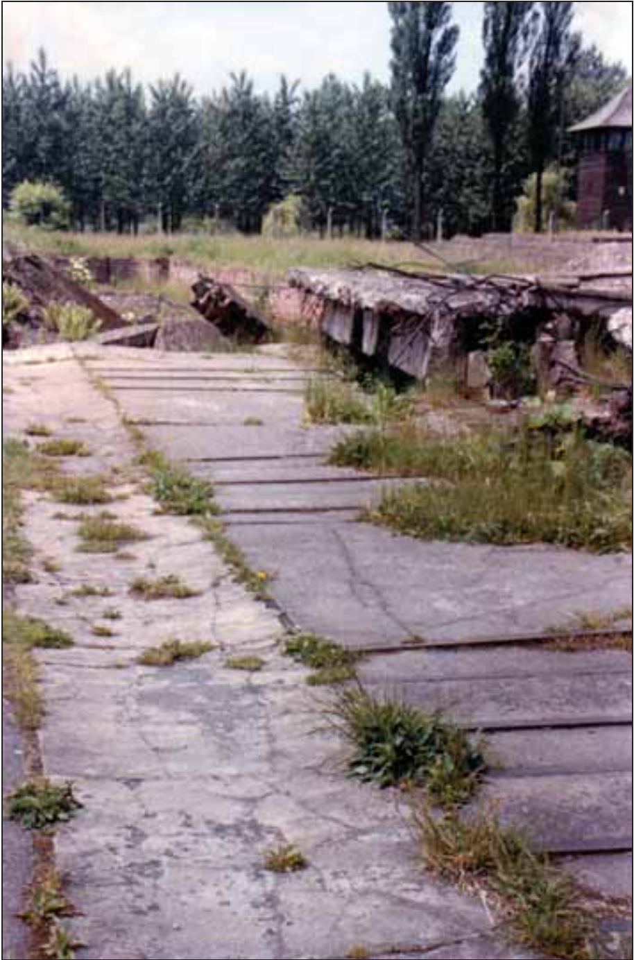
Photograph 219: as Photo 216; rails for the corpse-introduction cart to the first three furnaces and location of the transverse rails for the turntable (direction east-west).
