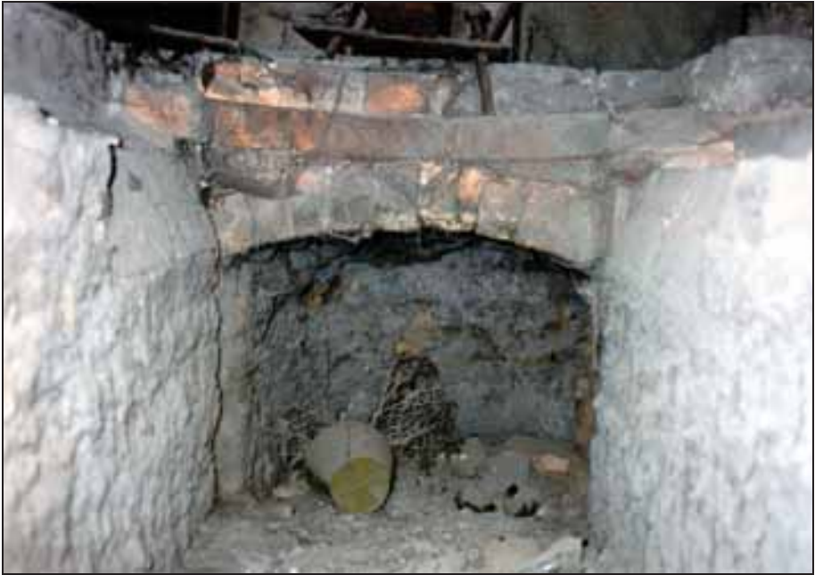
Photograph 102: Ruins of furnace no. 3: flue-duct opening of the left-hand muffle.
