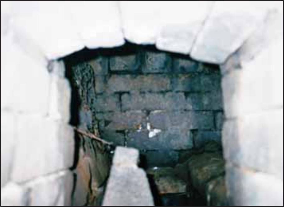
Photograph 281: as above. View into the auxiliary gasifier. Background: the wall of the muffle's ash chamber. Foreground: the end of an iron bar from the auxiliary hearth grate.
