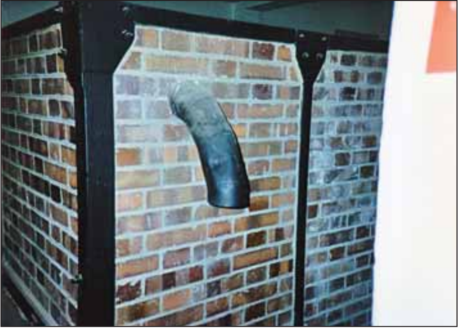
Photograph 76: Air pipe originally connected to a blower.
