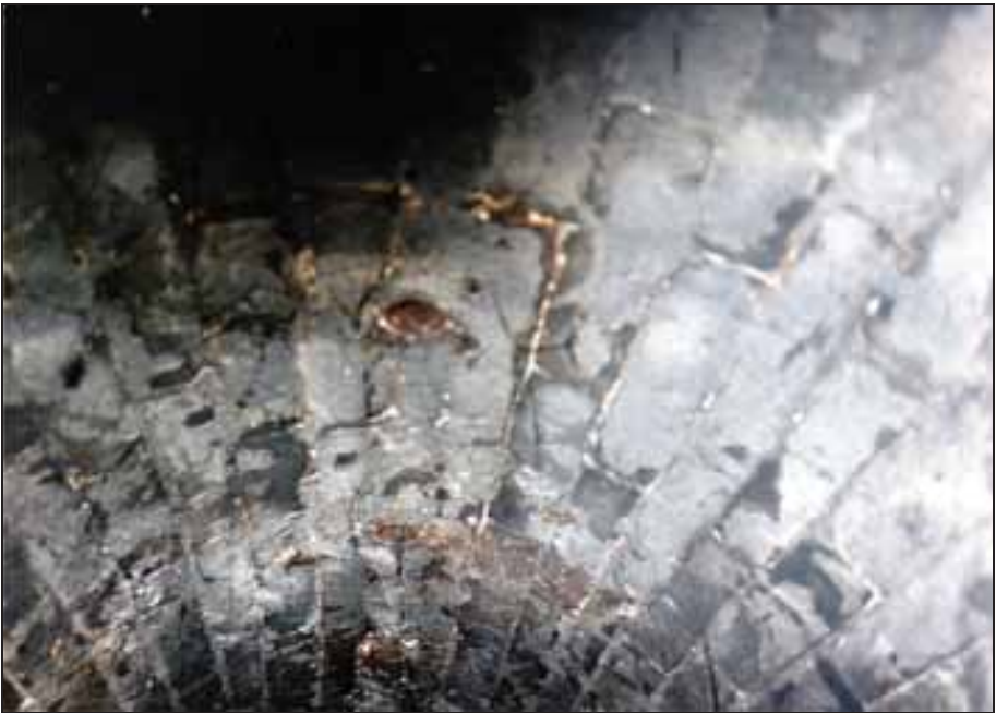
Photograph 61: Vaulted ceiling of the right-hand muffle; outlets of pipes connected to the blower.
