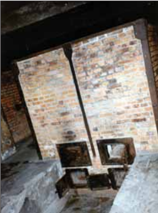
Photograph 97: Furnace no. 1, rear side. The furnaces were reconstructed without gasifiers. The gasifiers' coke-loading doors are therefore necessarily in the wrong position over those of the ash-chamber doors. See Photo 78.
