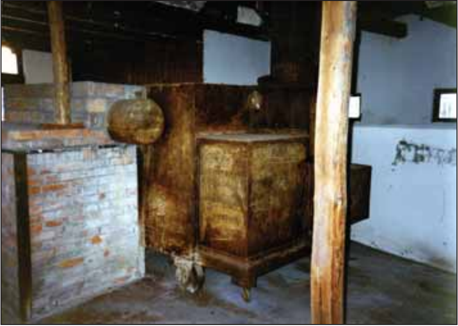
Photograph 45: Rear of the furnace, right-hand side. At the top of the gasifier, the rear part of the original oil tank sticks out, which was recklessly walled-in. The furnace's original body is mounted on metal wheels.
