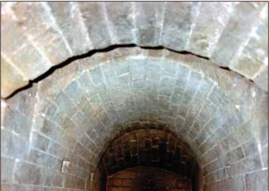
Photograph 321: as above; the vaulted muffle ceiling with the smoke-duct opening in the foreground.
