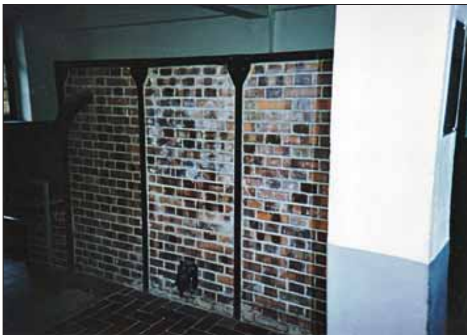
Photograph 73: Left side of the furnace: Door of the combustion-air-intake channel leading into the ash chamber of the left-hand muffle.
