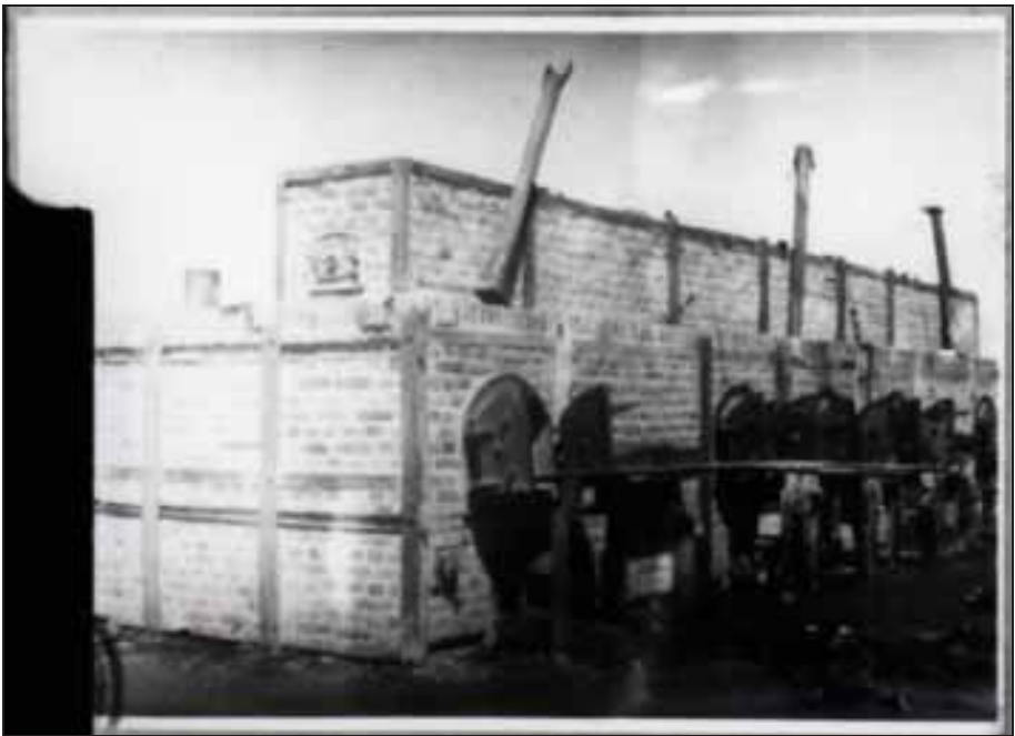
Photograph 286b: as above; the furnaces.
