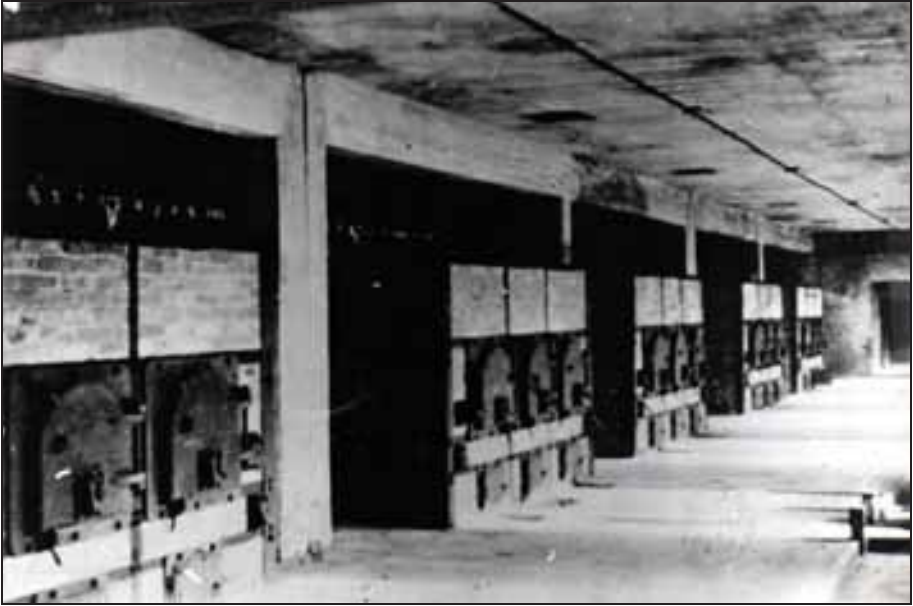
Photograph 115: SS photo of the TOPF coke-fired triple-muffle furnaces at Crematorium II at Birkenau. APMO, microfilm no. 290.
