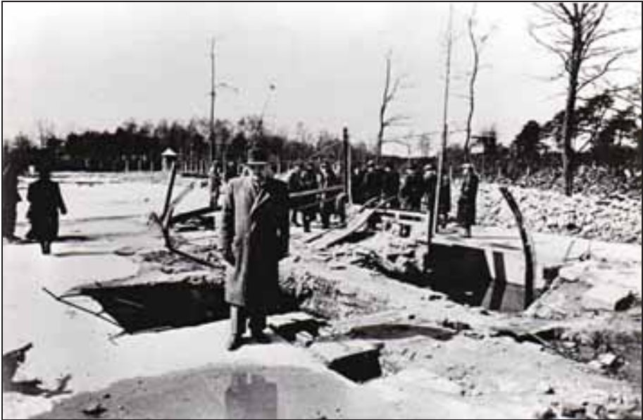
Photograph 222: Ruins of Crematorium V. Wrought-iron frame of the TOPF eight-muffle furnace and service pit. Polish photo of May 1945. APMO, negative no. 21334/141.
