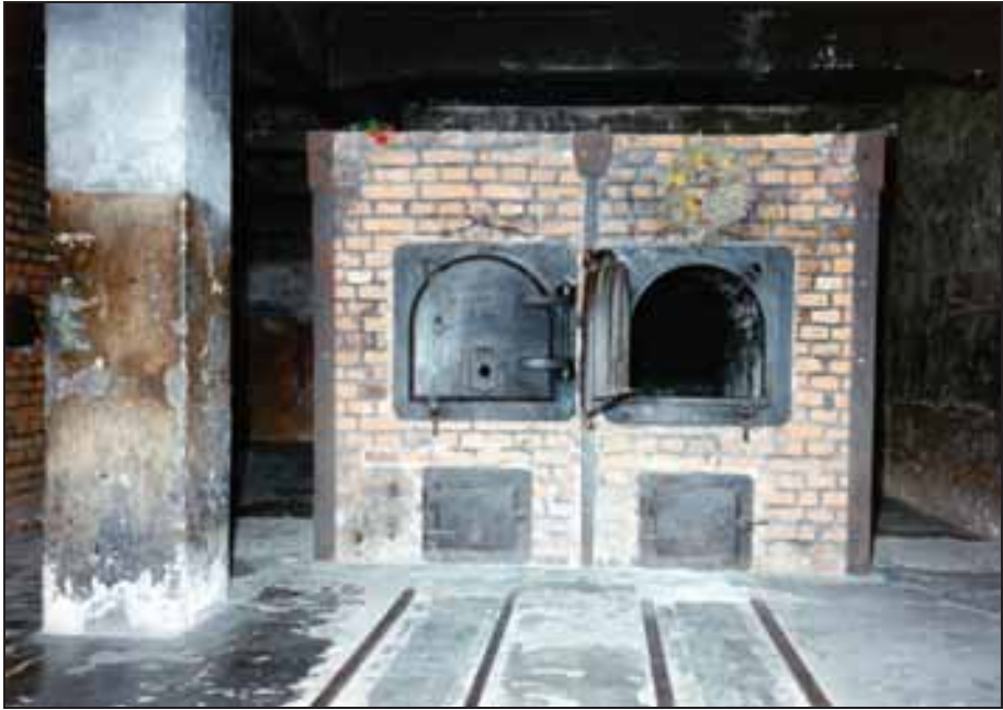
Photograph 90: Furnace no. 2. The reconstruction omitted the transverse anchor bars and the combustion-air-intake channels next to the muffle doors; in addition, the muffle doors were reversed. Compare Photo 51.
