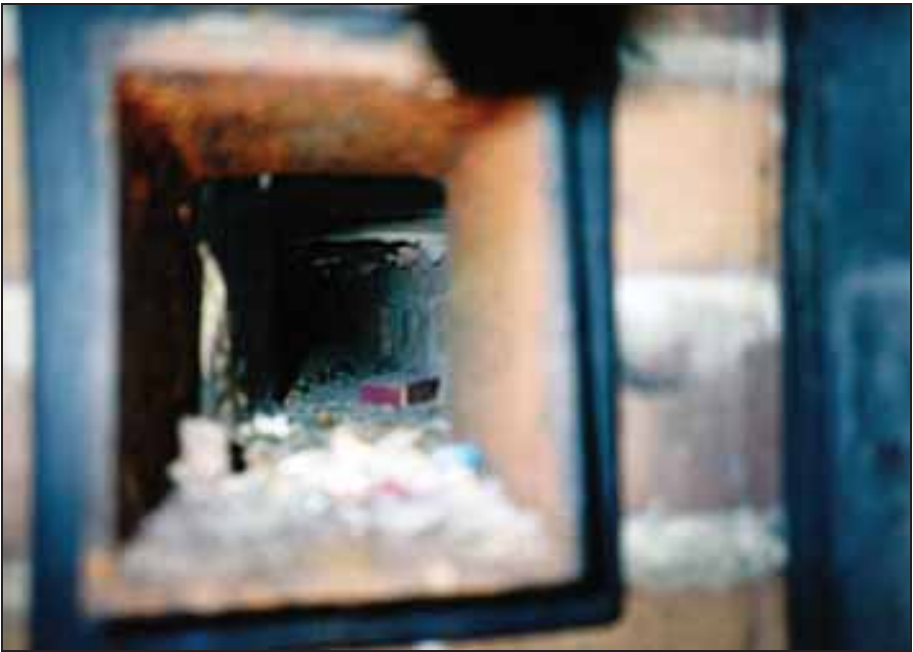
Photograph 57: Combustion-air channel of the left-hand muffle, closed with the door visible in the next photograph.
