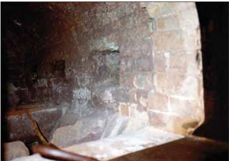
Photograph 138: as above, rectangular inter-muffle openings in the right-hand muffle wall.
