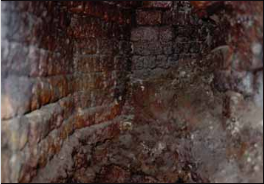
Photograph 315: Inside of the gasifier of the TOPF furnace at the Gusen concentration camp. The refractory lining shows extensive fusion.
