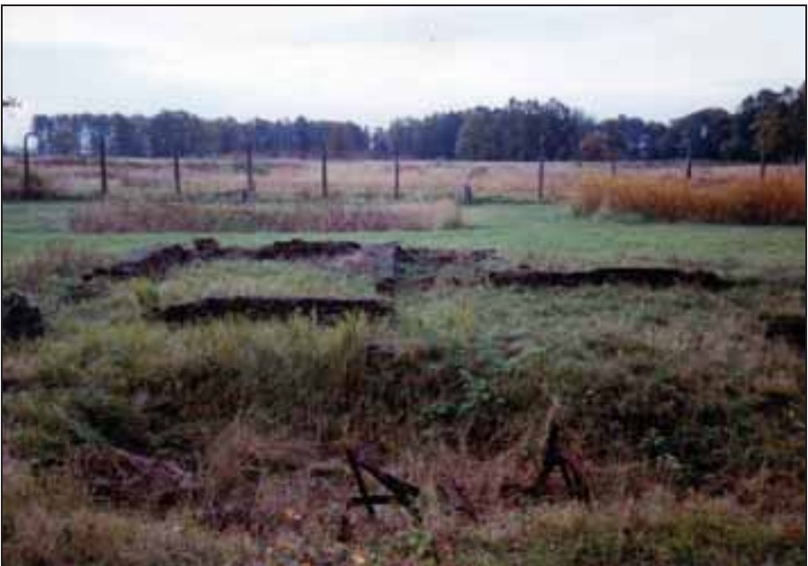
Photograph 235: as above. Framework fragments of the TOPF eight-muffle furnace in the foreground (direction north-south).
