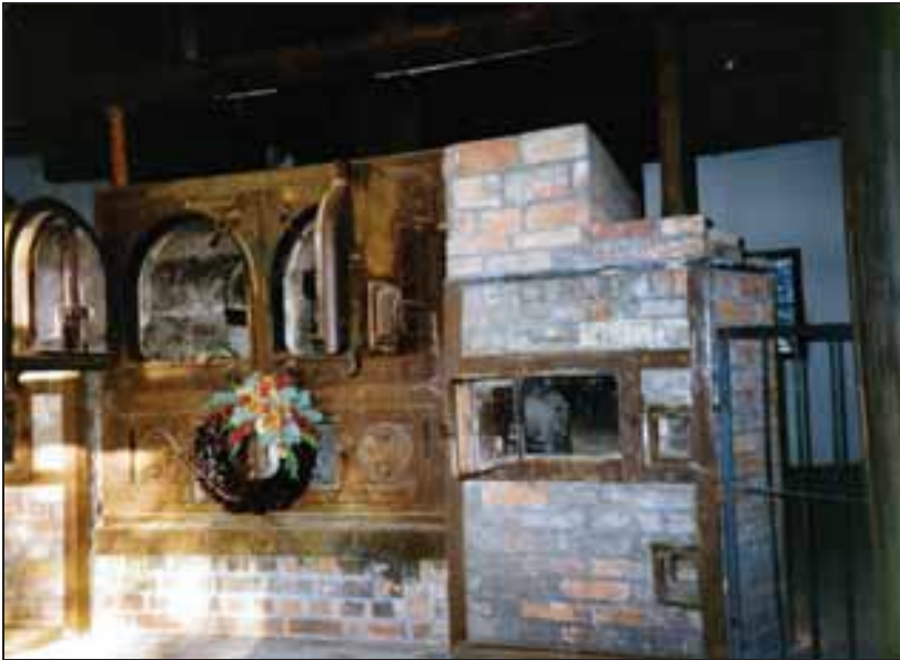
Photograph 38: Original furnace body with right-hand masonry gasifier.
