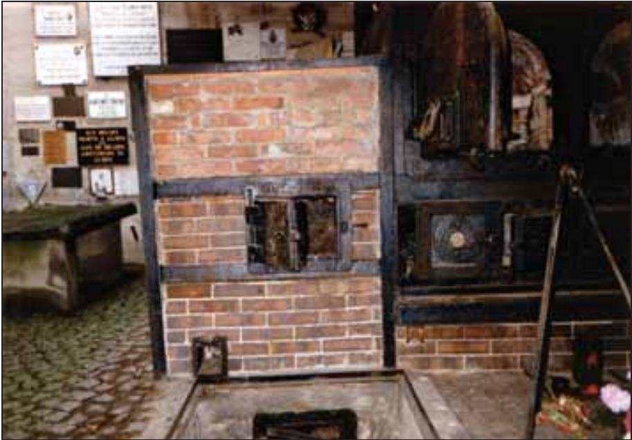
Photograph 4: The furnace's left-hand gasifier with coke-loading door and the gasifier's primary air-intake door (with the shutter missing).
