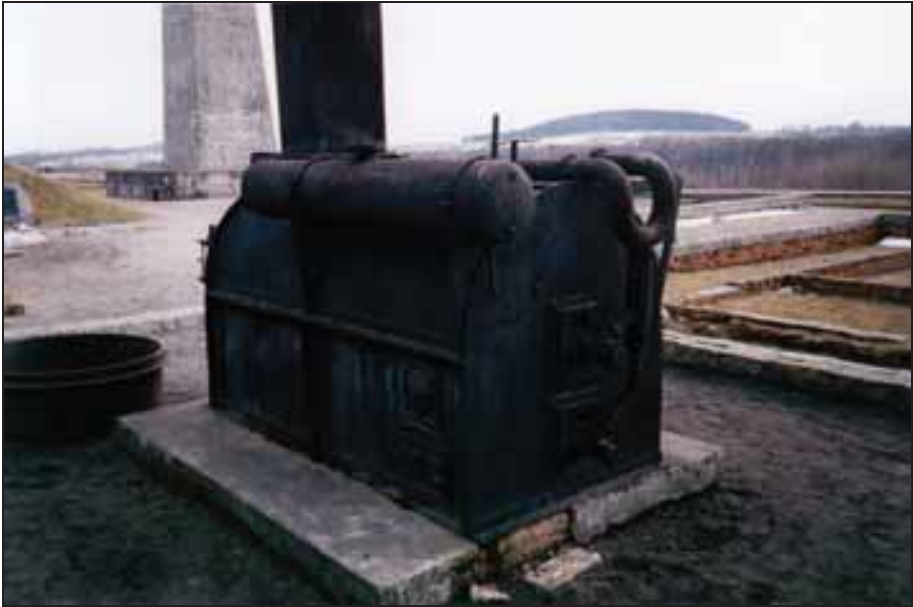
Photograph 333a: rear view. Left-hand side: naphtha tank; below it: combustion-air inlet and access door; right-hand side: combustion-air pipes; rear end: main (top) and auxiliary burner (bottom).
