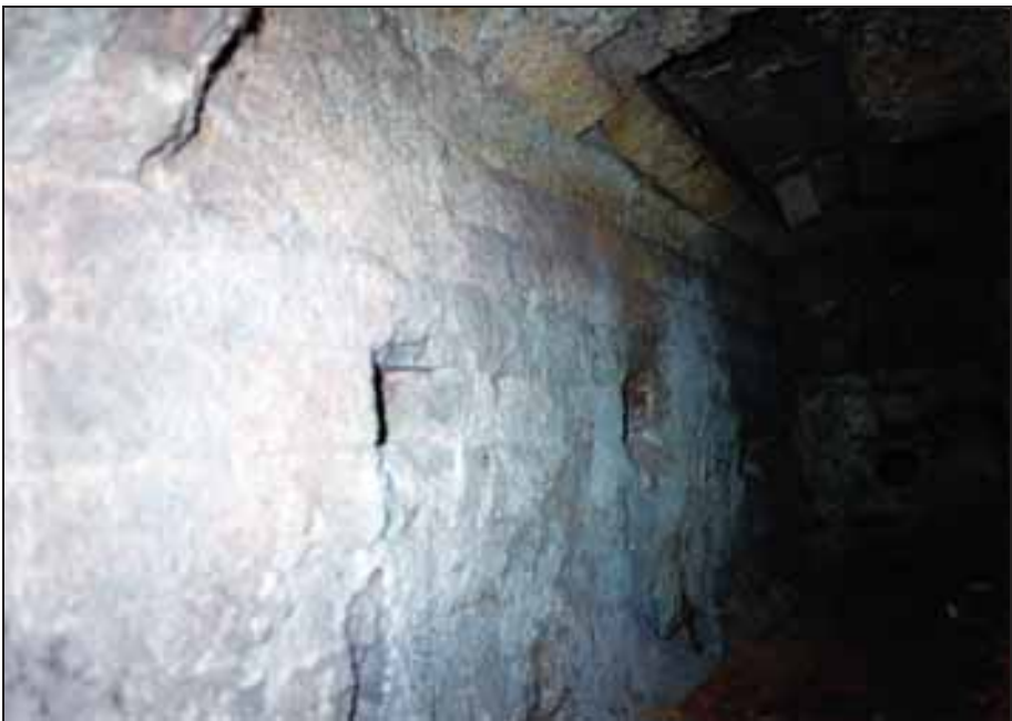
Photograph 241; as above, close-up of combustion-air-supply holes.
