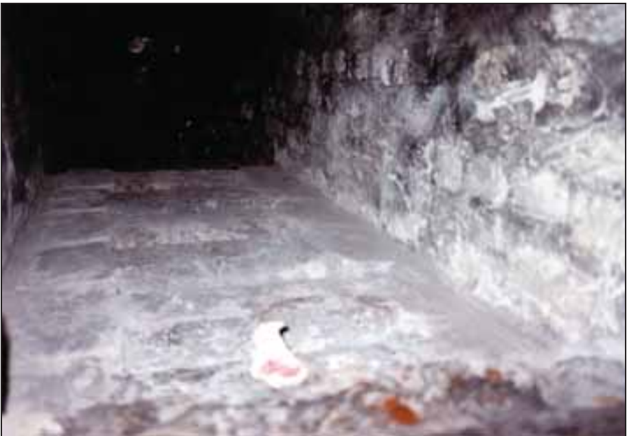
Photograph 93: Furnace no. 2: grate of the left-hand muffle.
