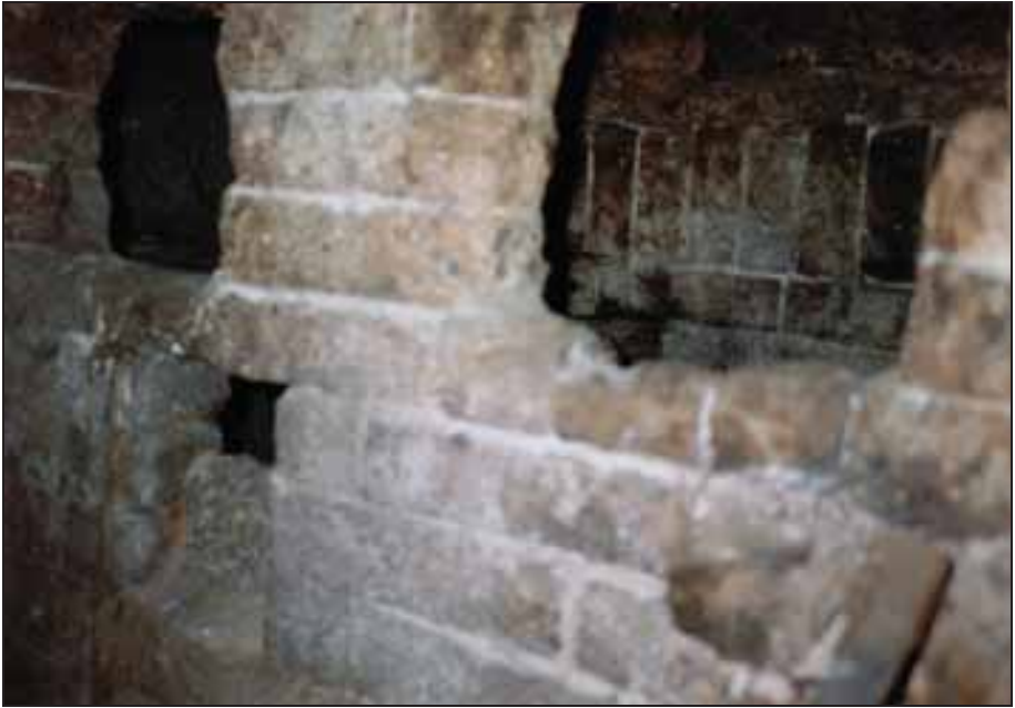
Photograph 20: Left-hand muffle: partition wall with inter-muffle openings.
