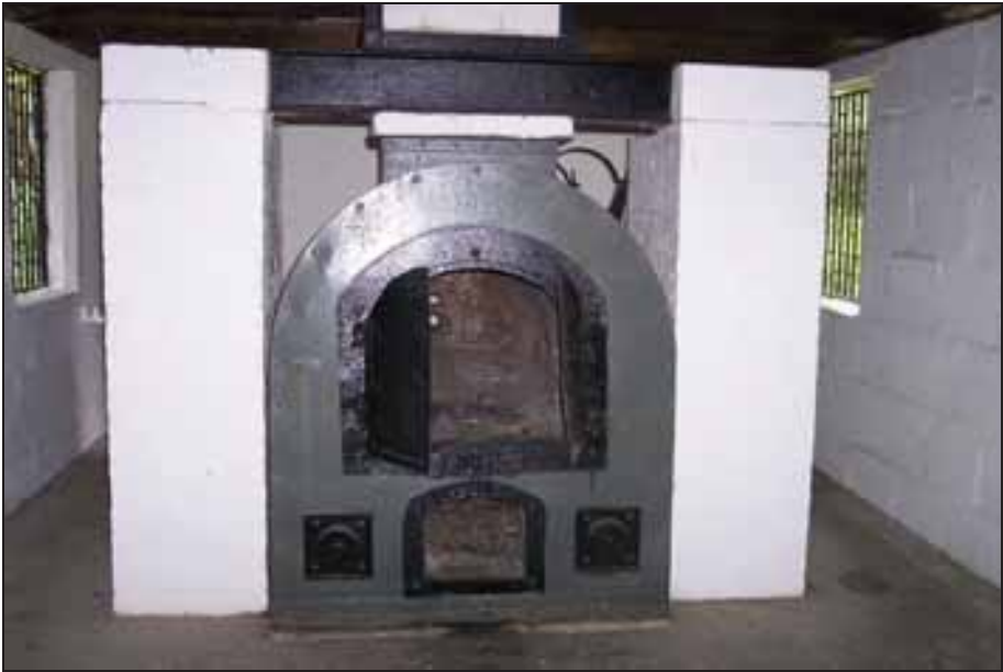
Photograph 331a: Naphtha-fired cremation furnace at Blechhammer sub-camp.
