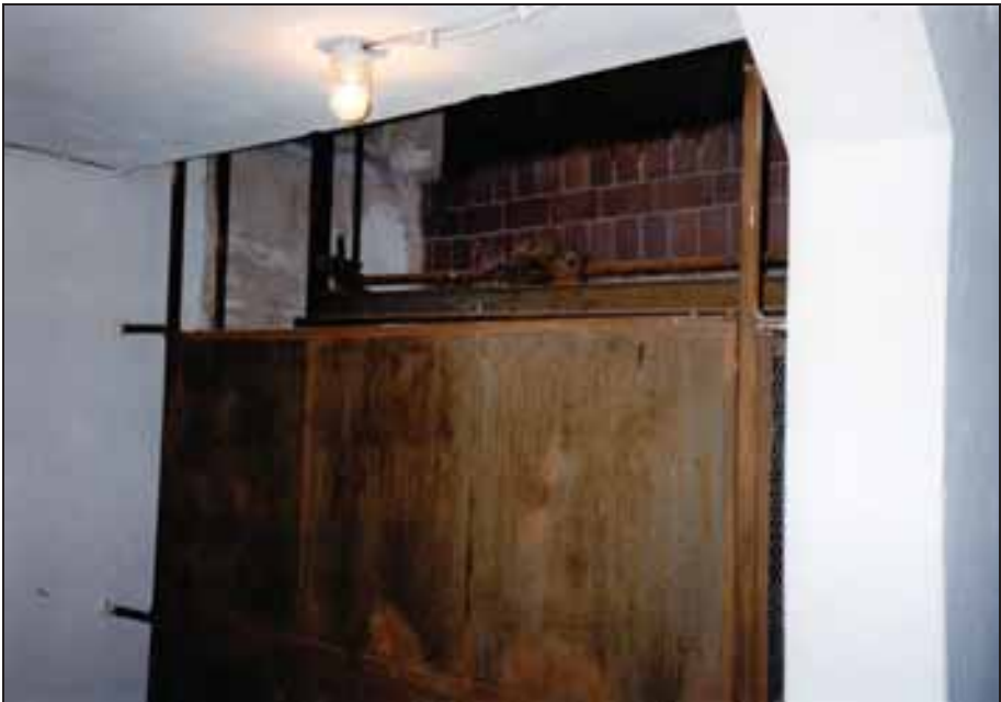
Photograph 213: as above, rear.
