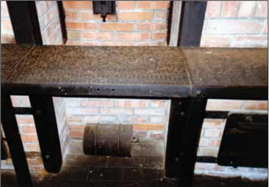
Photograph 172: as above; cement counter weight of the smoke-duct damper.
