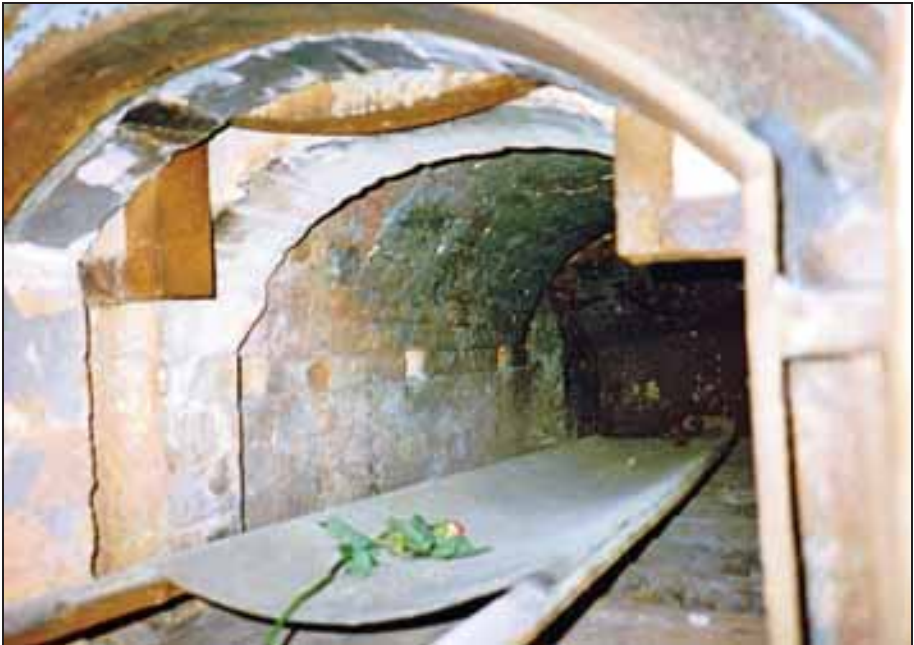
Photograph 253: Second furnace, inside the muffle; left-hand side with three opening for combustion-air supply.
