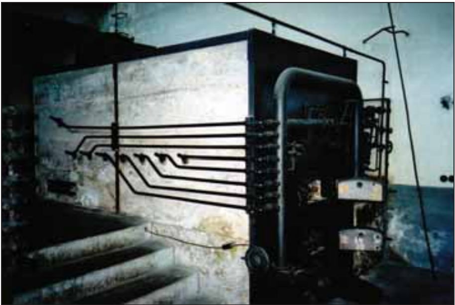
Photograph 347: as above; left-hand side and rear of the furnace.
