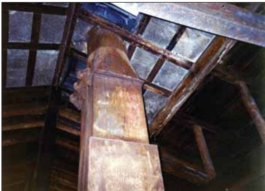
Photograph 49: Top part of the chimney.
