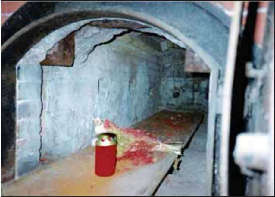
Photograph 240: as above; left-hand muffle wall with opening for the combustion-air supply.
