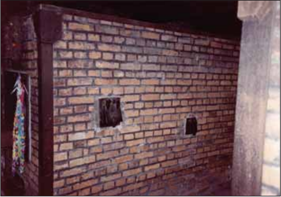
Photograph 96: Furnace no. 1, right-hand side. Original doors of combustion-air channels. The Polish reconstructions did not include those channels. The number, type and position of the doors are also wrong. The larger door originally belonged to an eight-muffle furnace, and the smaller door was located lower. Cf. Photo 73.
