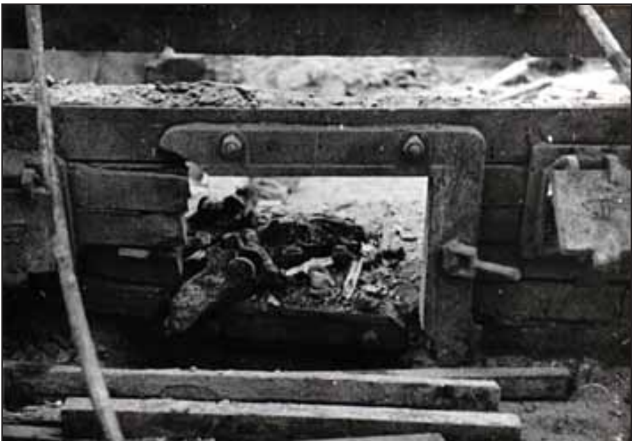
Photograph 227: as above, ash chamber's door frame of the muffle located in the north-western corner. Visible on the right is the door of the ash chamber's combus- tion-air channel.
