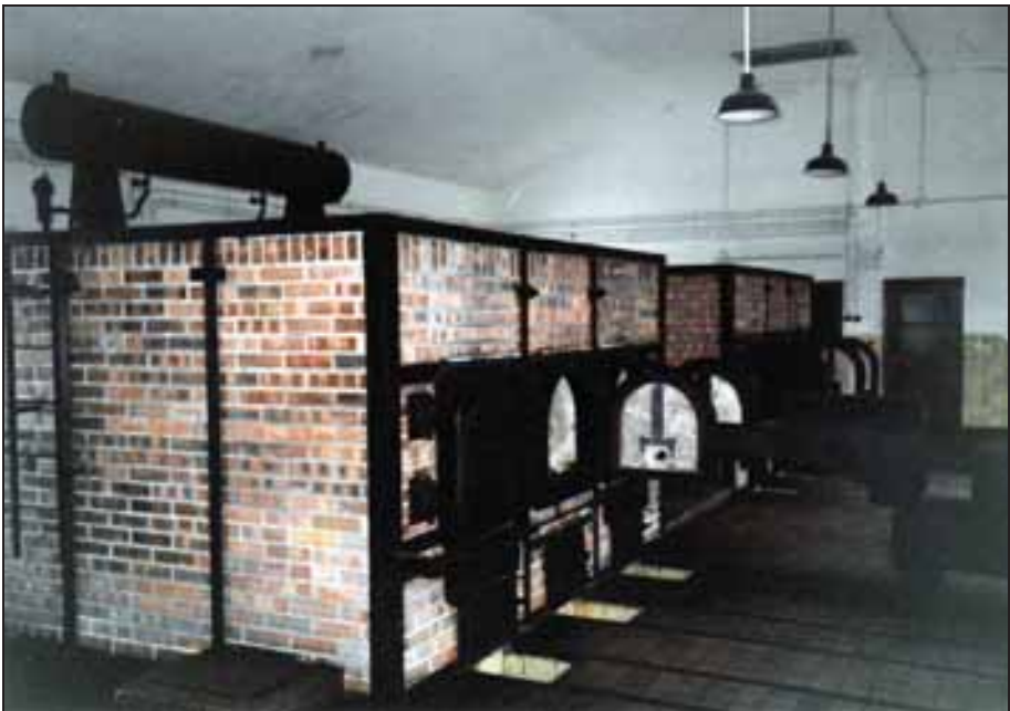
Photograph 114: TOPF triple-muffle cremation furnaces in the Crematorium at Buchenwald Concentration Camp.
