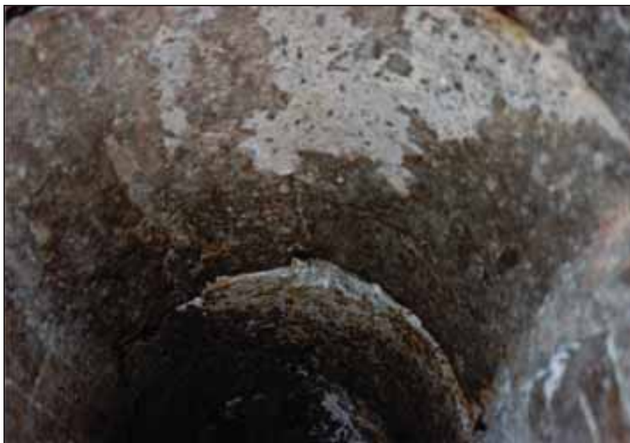
Photograph 26: Right-hand muffle: Vaulted muffle ceiling with the outlet of one of the pipes connected to a blower.
