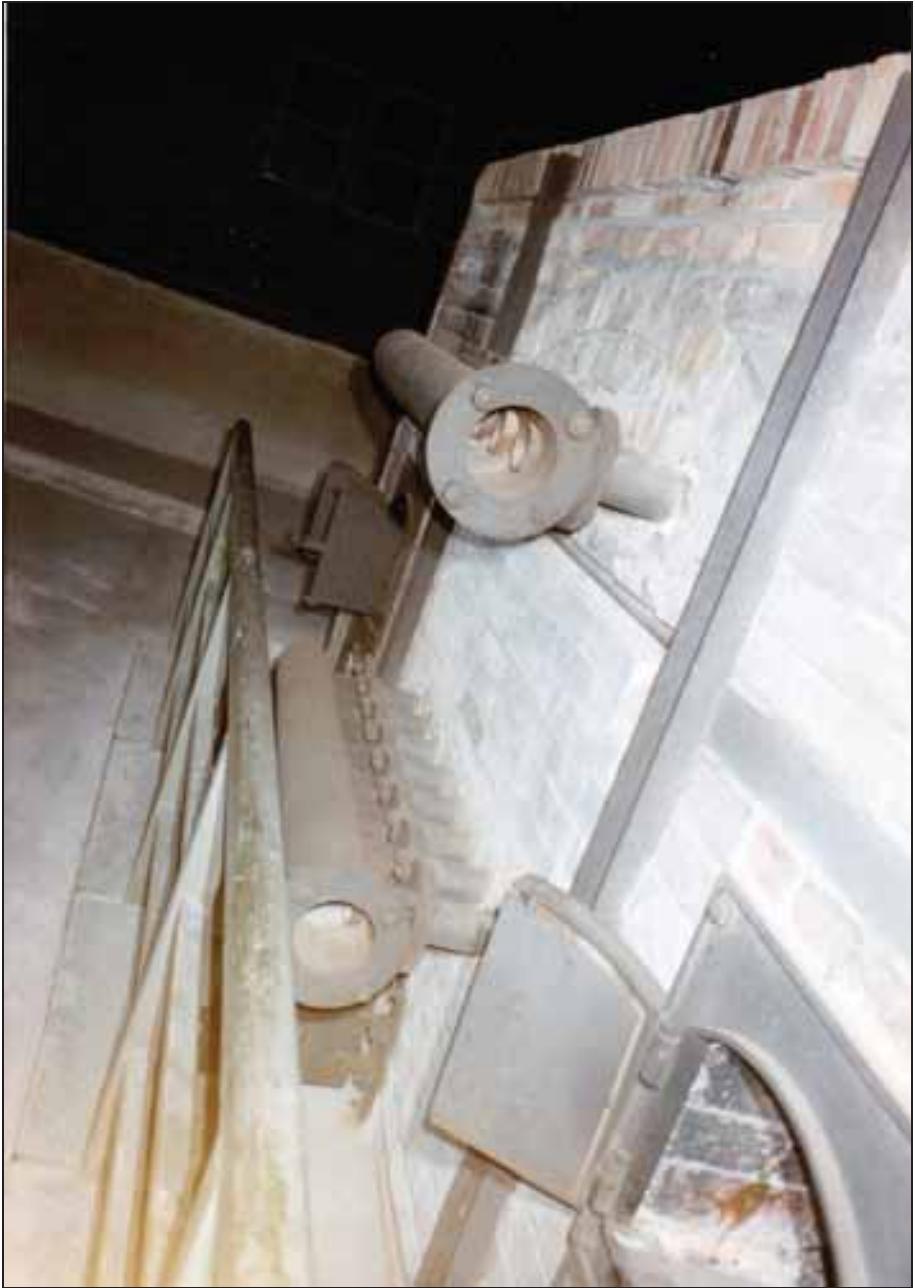
Photograph 308: as above. Hot-water pipes of the recuperator.
