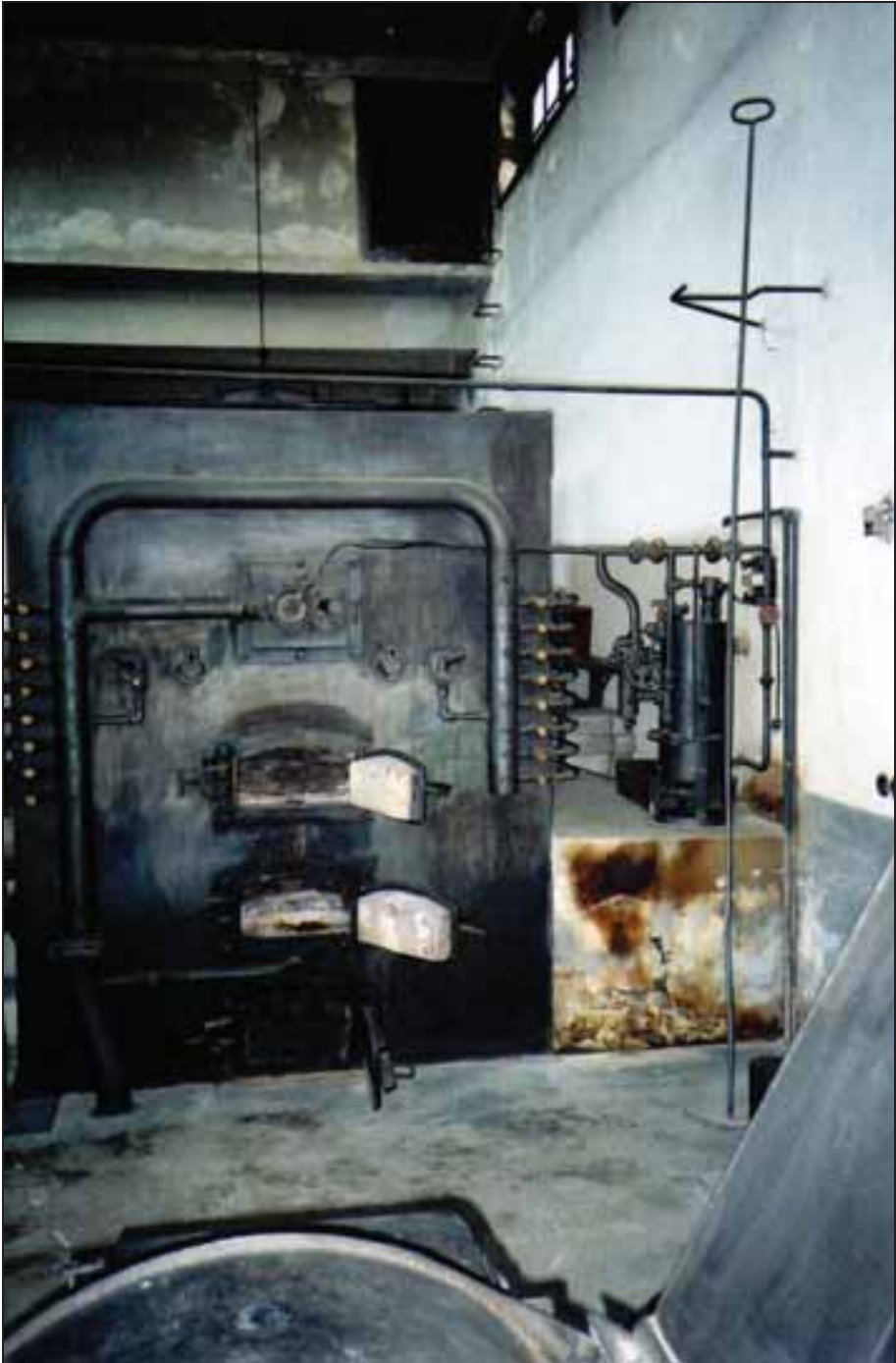
Photograph 349: as above; on the right, next to the wall, is the naphtha preheater behind a long scraper.
