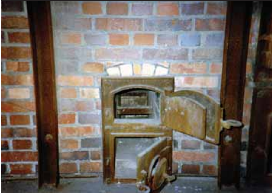
Photograph 260: First furnace, the auxiliary gasifier's service doors: loading door (top) and ash-chamber door (bottom).
