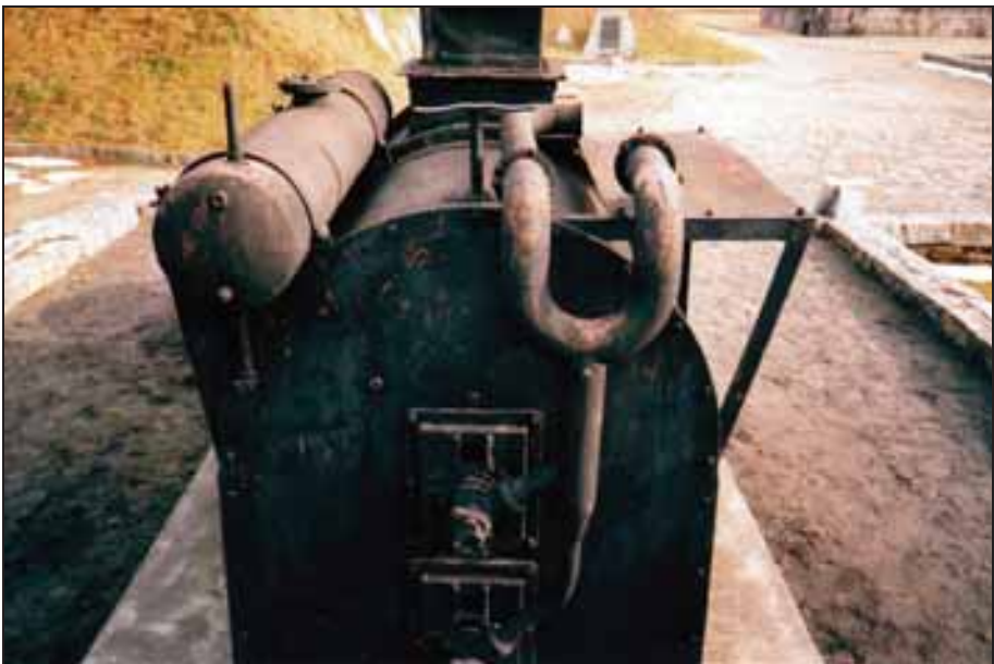
Photograph 333b: as above. The air pipes were originally connected to a blower installed on the shelf to the right.
