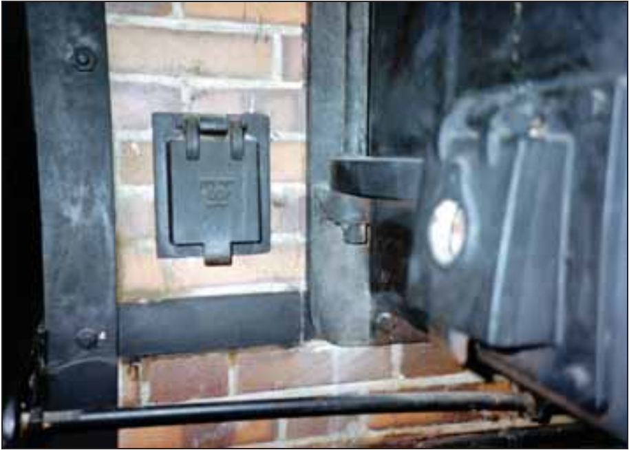
Photograph 58: Door for the combustion-air channel of the left-hand muffle.
