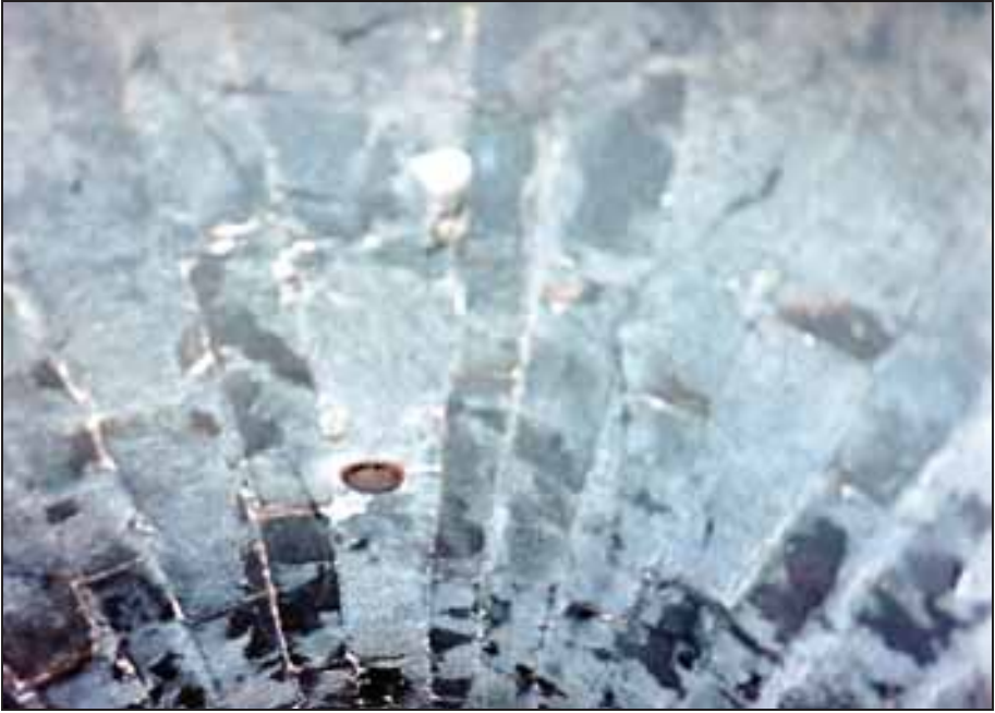
Photograph 60: Vaulted ceiling of the left-hand muffle; outlets of pipes connected to the blower.
