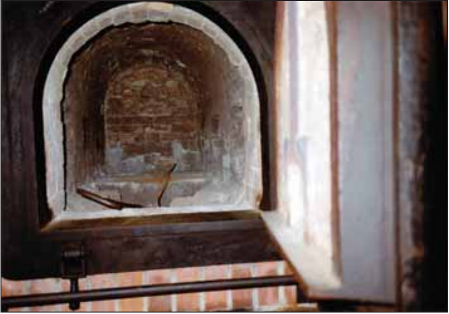
Photograph 135: as above, central muffle. Both side walls have three rectangular openings connecting it to the side muffles.
