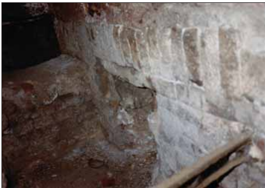
Photograph 27: Right-hand muffle: ash compartment with an opening connecting it to the gasifier.
