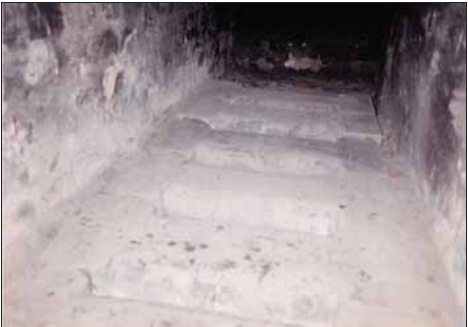
Photograph 95: as above; grate of the right-hand muffle.
