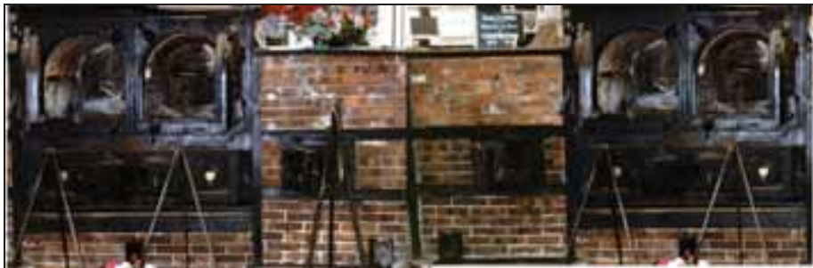
Document 241: Composite photograph based on the TOPF double-muffle cremation furnace at the Gusen camp illustrating the structure of the Topf eight-muffle furnace.
