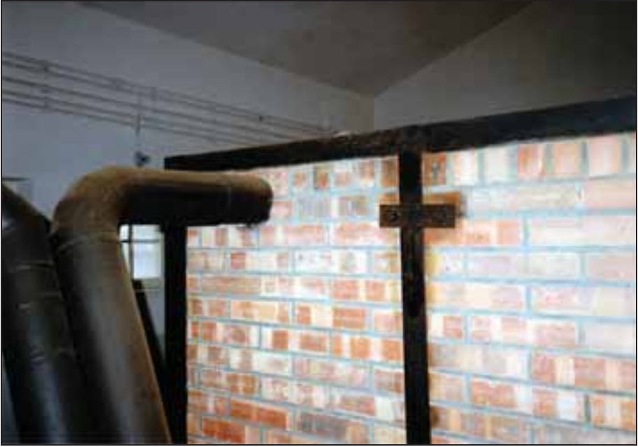
Photograph 193: Blower tube connected to the coke-fired furnace.
