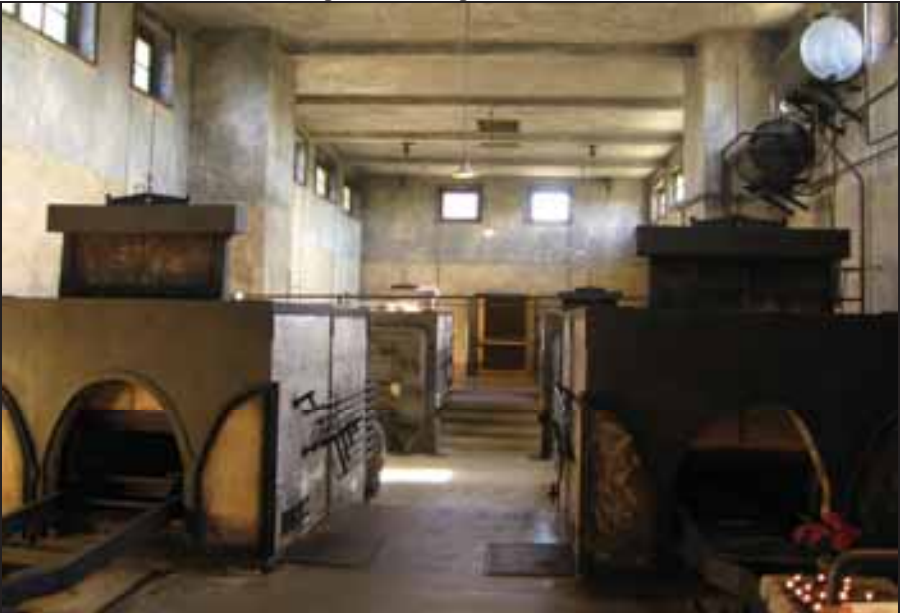
Photograph 345a: as above, viewed from eye level.
