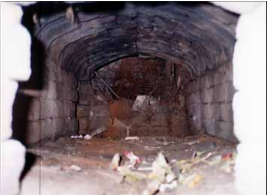
Photograph 273: The ash chamber of the left-hand muffle. Top: underside of the muffle's grate bars. On the left wall: opening connecting it with the auxiliary hearth. At the back: the gasifier's pit.
