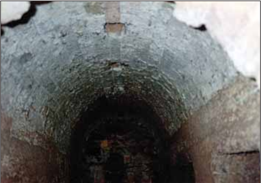
Photograph 132: as above; the apex of the vaulted ceiling sports four square openings which open into tubes supplying the muffle with combustion air.
