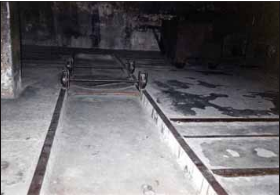
Photograph 105: Transverse rails and rotating platform (turntable).
