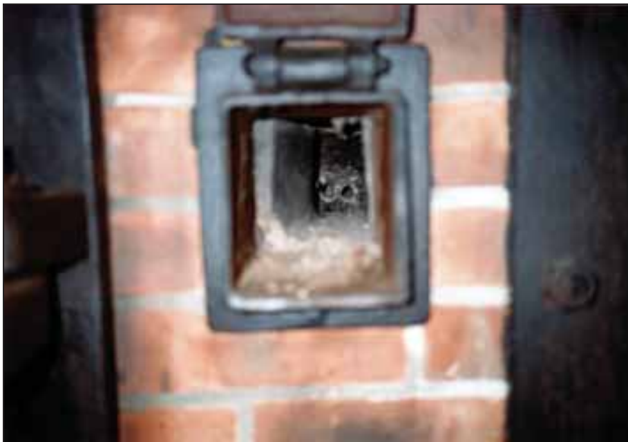
Photograph 149: as above, the muffle's combustion-air-supply channel.
