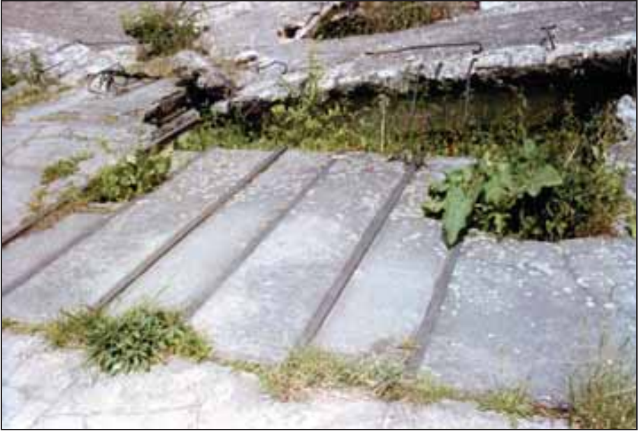
Photograph 217: as above; rails for the corpse-introduction cart.
