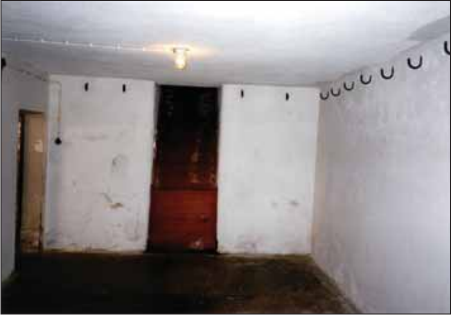
Photograph 210: as above; basement morgue, wooden corpse chute.
