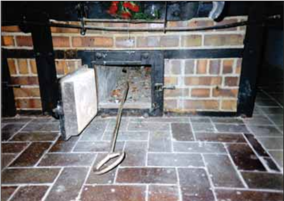
Photograph 71: Ash chamber of the right-hand muffle.
