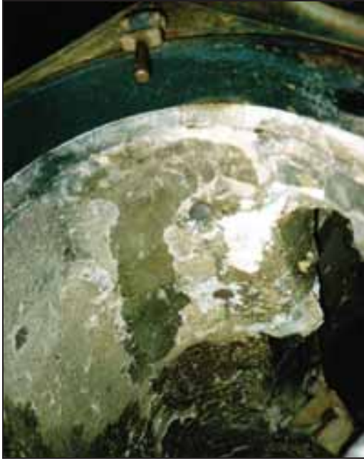
Photograph 41: Vaulted ceiling of the left-hand muffle; to the right: outlets of pipes connected to the blower.
