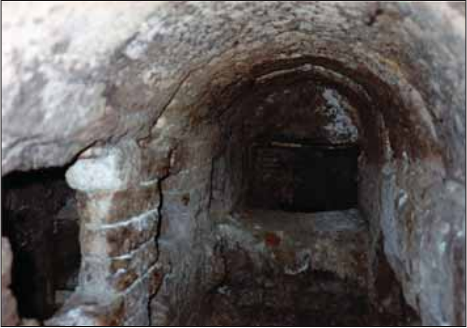
Photograph 22: Right-hand muffle: to the left the partition wall with three inter-muffle openings.
