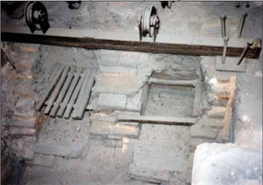
Photograph 101: as above, seen from the rear: original grate of the left-hand gasifier and the two transverse support bars of the right-hand grate. The bar with the rollers, originally attached to the ceiling, was used to operate the furnace's two flue dampers.
