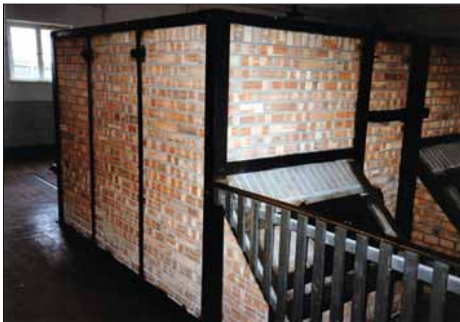
Photograph 126: as above, left-hand rear view. with coke-loading door of the gasifier.
