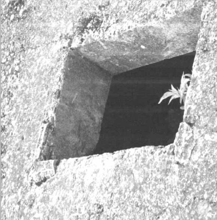
III. 12: Ceiling of the furnace room of Crematorium III. First ventilation opening (seen from the west). © Carlo Mattogno
