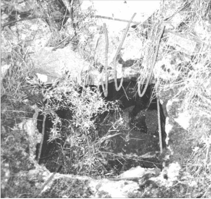
III. 25: Concrete roof of morgue 1 of Crematorium II in Birkenau. Provan's opening 7 in October 1991. © Carlo Mattogno
