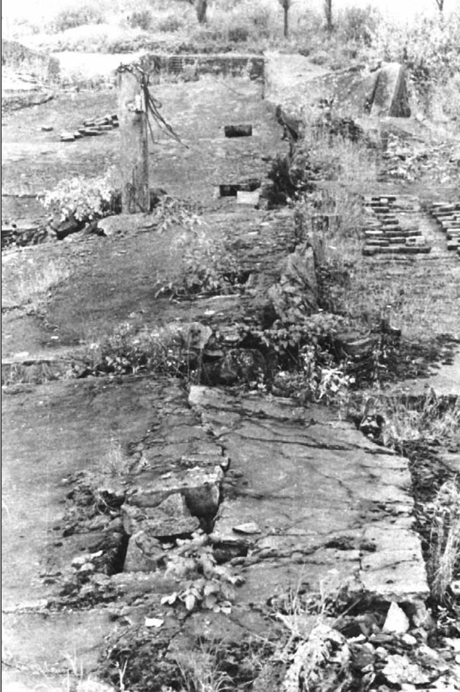
III. 14: All five ventilation openings of the ceiling of the furnace room of Crematorium III. Photo by J.-C. Pressac.
