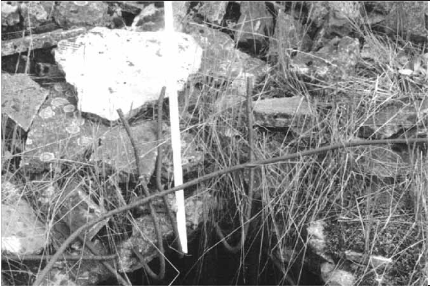
III. 24: Concrete roof of morgue 1 of Crematorium II in Birkenau. Reinforcement bars of Provan's opening 7 in June 1990. © Carlo Mattogno
