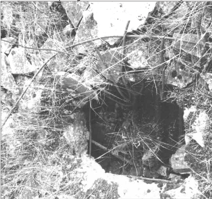
III. 26: Concrete roof of morgue 1 of Crematorium II in Birkenau. Provan's opening 7 in July 1992. © Carlo Mattogno
