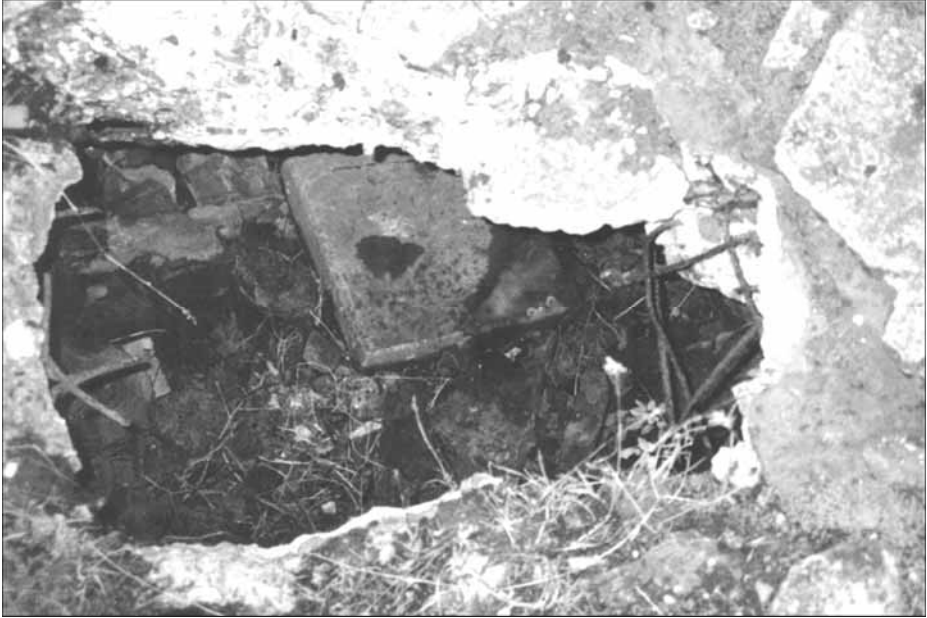
III. 29: Concrete roof of morgue 1 of Crematorium II in Birkenau. Provan's opening 2 in October 1991. Inside the morgue on the floor a square concrete lid can be seen stemming from the sewer manhole of this crematorium. © Carlo Mattogno
