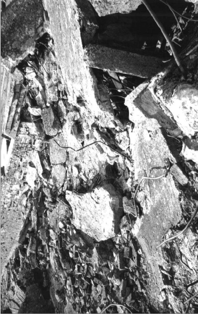
III. 9: Round opening for the pipe of the ventilation through the reinforced concrete roof of morgue 2 of Crematorium II in Birkenau. August 2000. © Carlo Mattogno.
