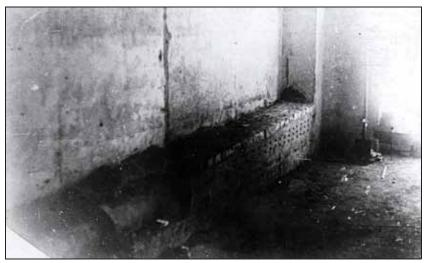
**Photo 10:** The interior of the disinfestation chamber at Stutthof, west wall: cast iron connection pipe to the oven located outside the delousing chamber and used to heat the air inside the chamber. Half of it is covered by perforated bricks.
