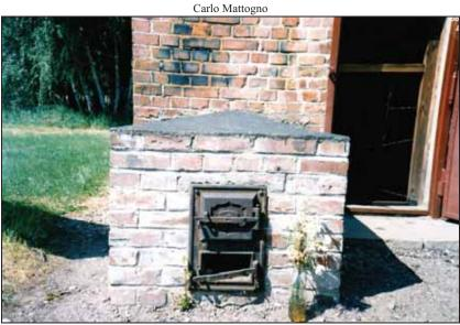
**Photo 6**: Delousing chamber at Stutthof, viewed from the south. The oven was used to heat the air inside the delousing chamber. Above: the fire door. Below: the ash door. © Carlo Mattogno
