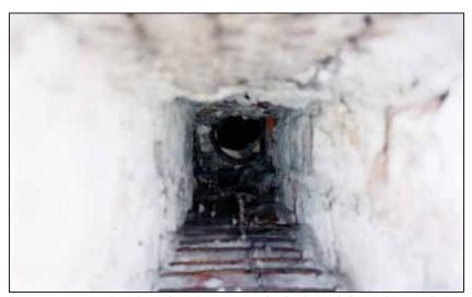
Photo 7: Delousing chamber at Stutthof, viewed from the south. The oven was used to heat the air inside the delousing chamber. Interior view of the combustion chamber. Beneath: the plane grid; above: the circular opening of the connection to the cast iron pipe located inside the delousing chamber. © Carlo Mattogno
