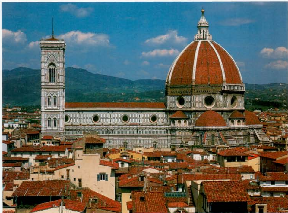
The dome of Florence Cathedral (1417–32) was the masterpiece of Brunelleschi, who studied Roman methods to enclose space on a huge scale, without support or even centering during construction.
