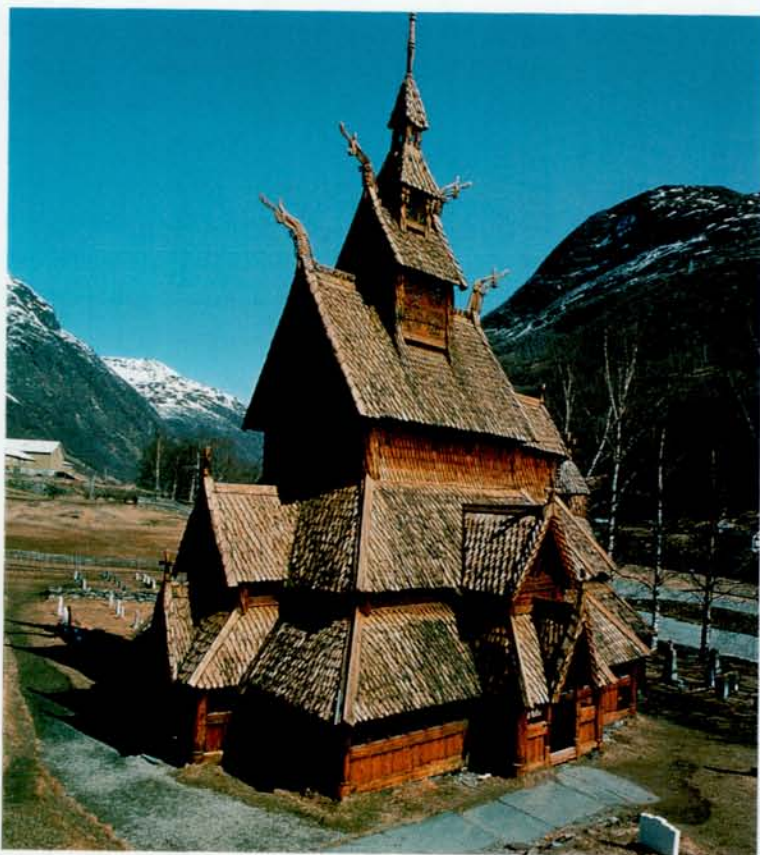
Stave Church of St Andrew at Borgund, Norway, is an outstanding illustration of Scandinavian carpentry using upright timbers. This twelfth-century example is one of twenty-eight to survive from over a thousand built.
