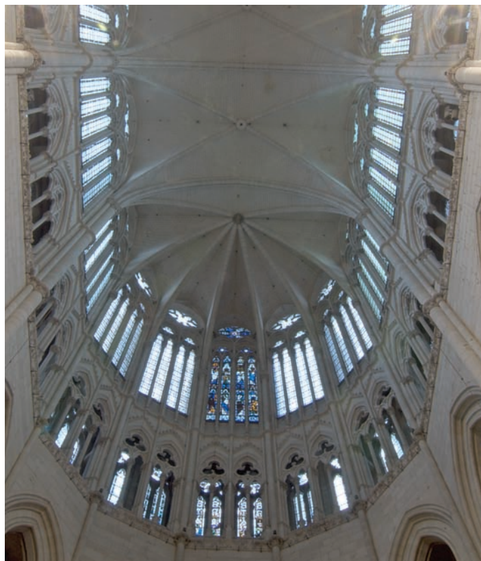
13-21 ROBERT DE LUZARCHES, THOMAS DE CORMONT, and RENAUD DE CORMONT, vaults, clerestory, and triforium of the choir of Amiens Cathedral, Amiens, France, begun 1220. ■◀
