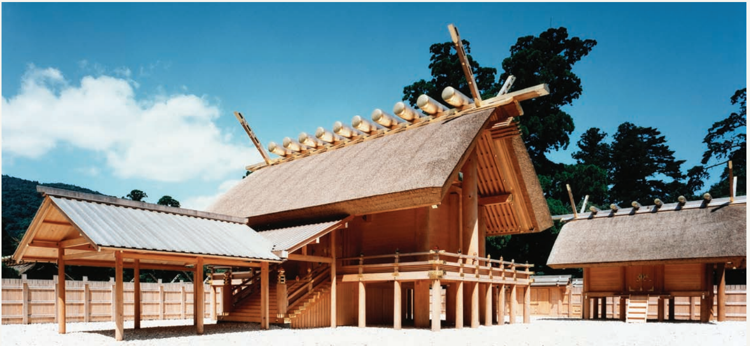
17-6 Main hall (looking northwest) of the Ise Jingu, Ise, Mie Prefecture, Japan, Kofun period or later; rebuilt in 1993.
