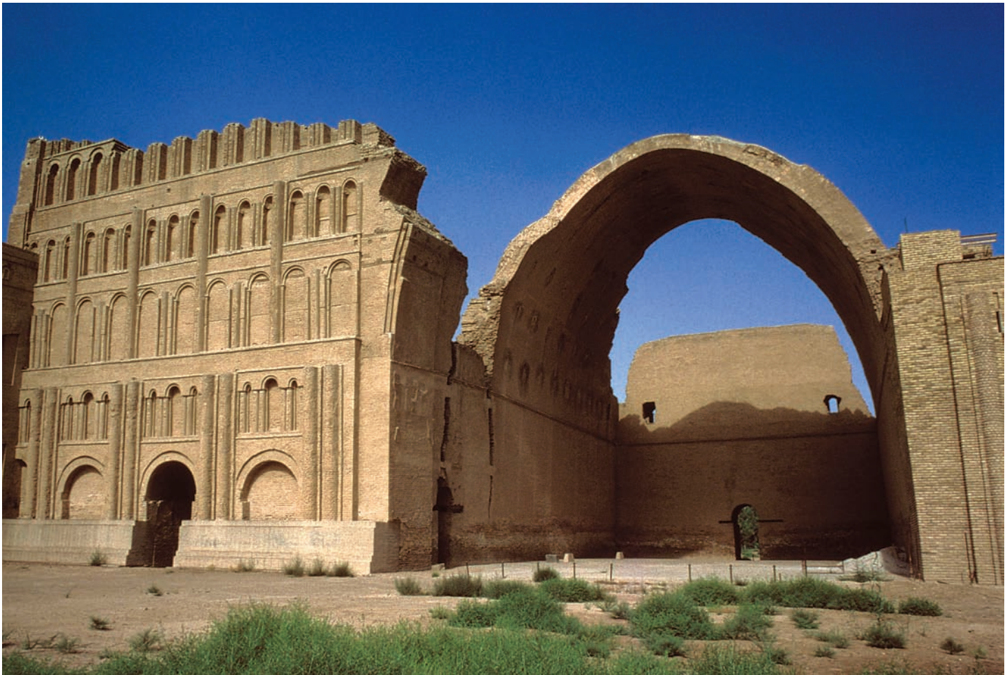
2-28 Palace of Shapur I, Ctesiphon, Iraq, ca. 250 CE.
