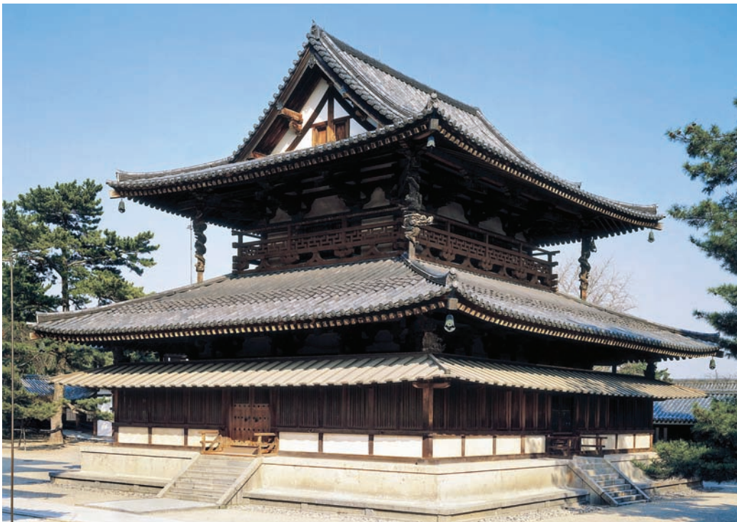
17-9 Kondo (looking southeast), Horyuji, Nara Prefecture, Japan, Nara period, ca. 680.
