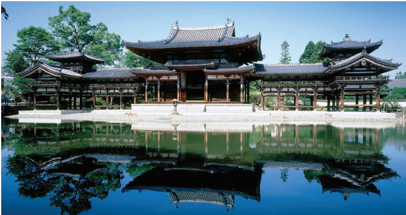
17-13 Phoenix Hall (looking west), Byodoin, Uji, Kyoto Prefecture, Japan, Heian period, 1053.
