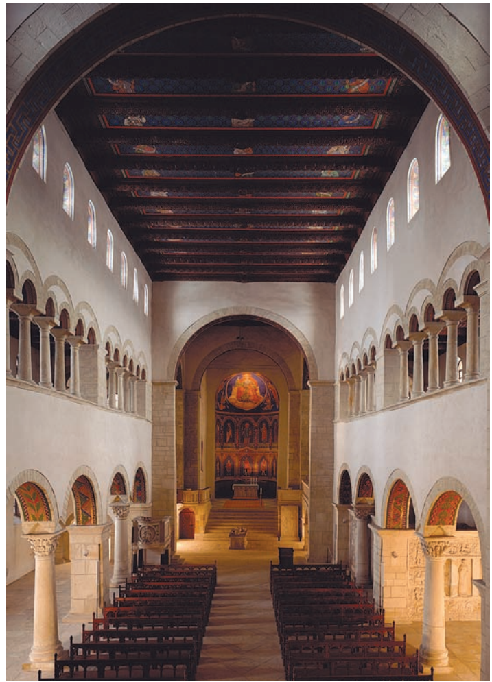
11-21 Nave of the church of Saint Cyriakus (looking east), Gernrode, Germany, 961–973.
