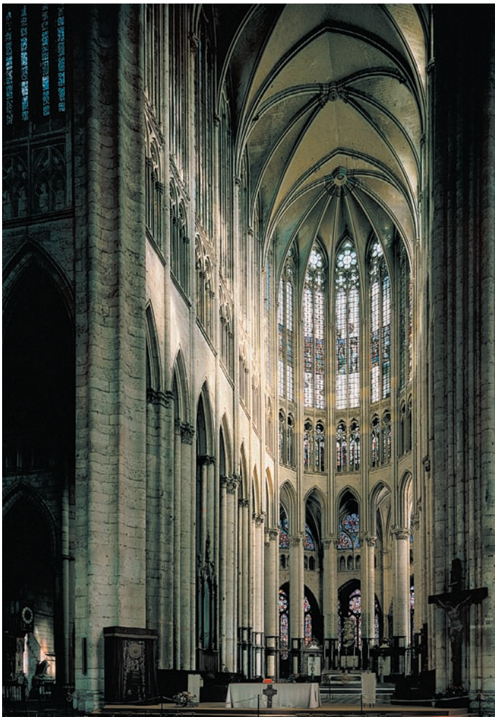
I-3 Choir of Beauvais Cathedral (looking east), Beauvais, France, rebuilt after 1284.
