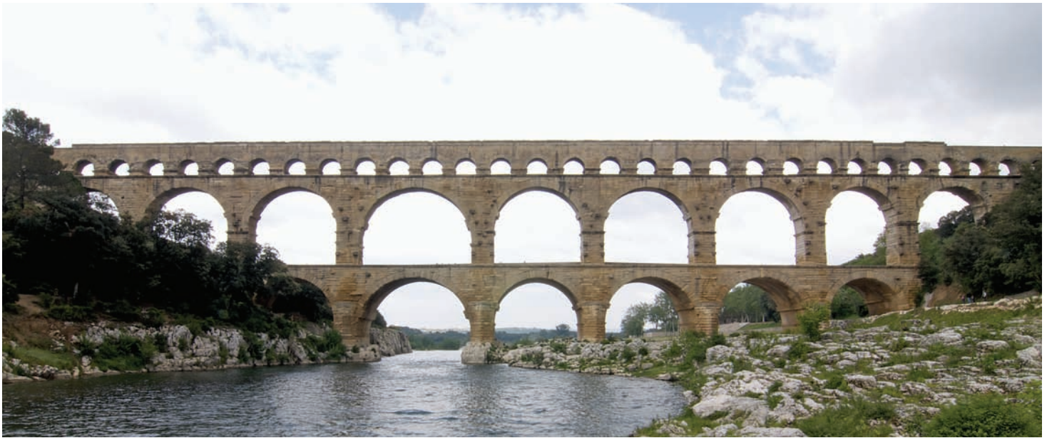
7-33 Pont-du-Gard, Nîmes, France, ca. 16 BCE. ■◀
