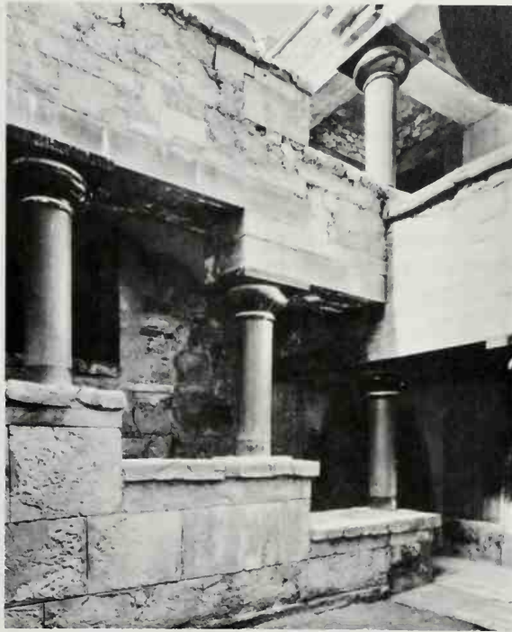
138. Staircase, east wing, Palace of Minos, Knossos, Crete. c. 1500 B.C.
