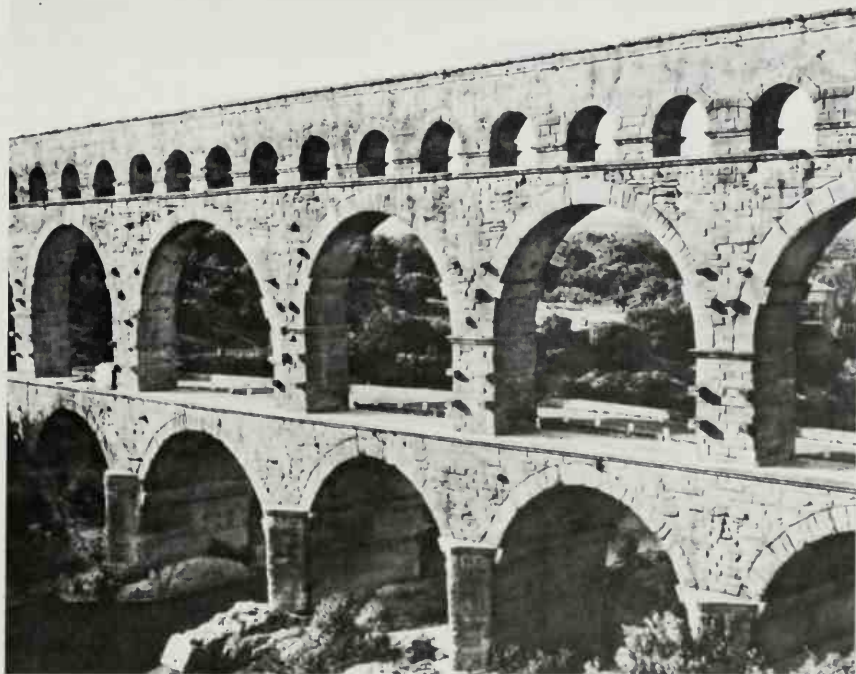
261. Pont du Gard, Nîmes, France. Early 1st century A.D.
