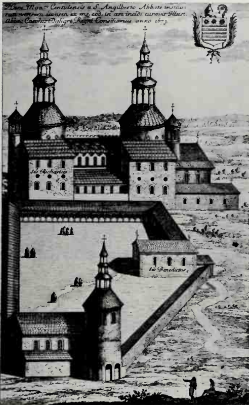
394. Abbey Church of St.-Riquier (engraved view by Petau, 1612, after an 11th-century manuscript illumination)
