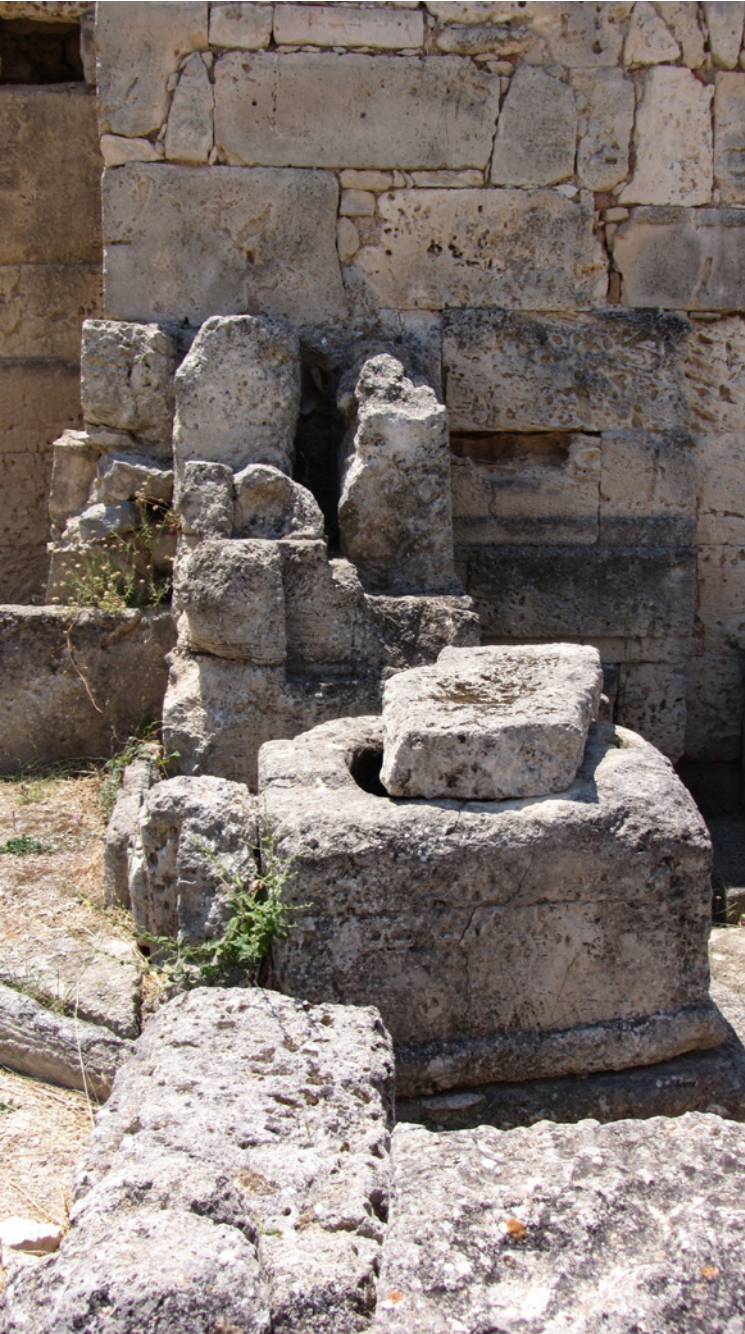
4. Cape Kolonna. Section of the north perimeter wall with a fountain/well. Photo credit: Irene Polinskaya
