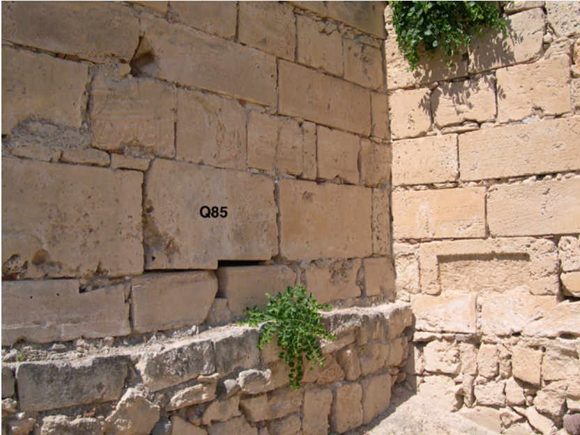
13. Cape Kolonna. North perimeter wall of Late Roman date with block Q85 from the Building with Inscribed Walls. Photo credit: Irene Polinskaya.
