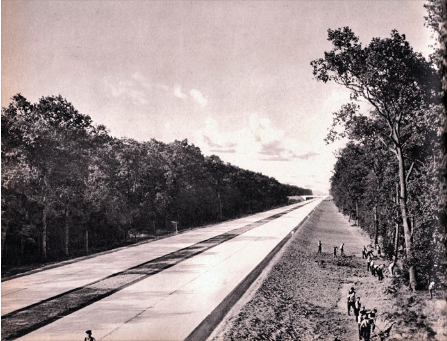
Figure 6.10. A Straight Stretch of Nearly Completed Autobahn
