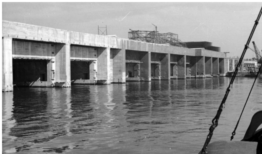
Figure 6.15. The Submarine Bunker at Saint-Nazaire, France
