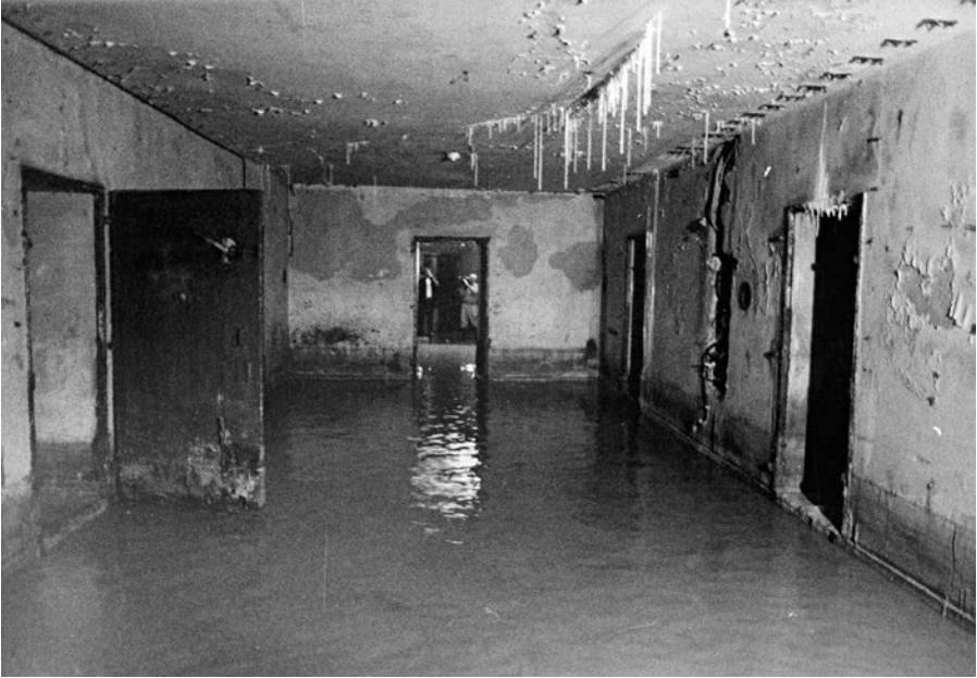
Figure E.1. The Flooded Führer Bunker in Berlin in 1990
