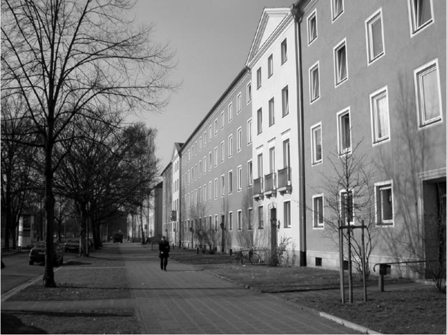
Figure 6.8. A Massive Four-Story Apartment Building in Nuremberg
