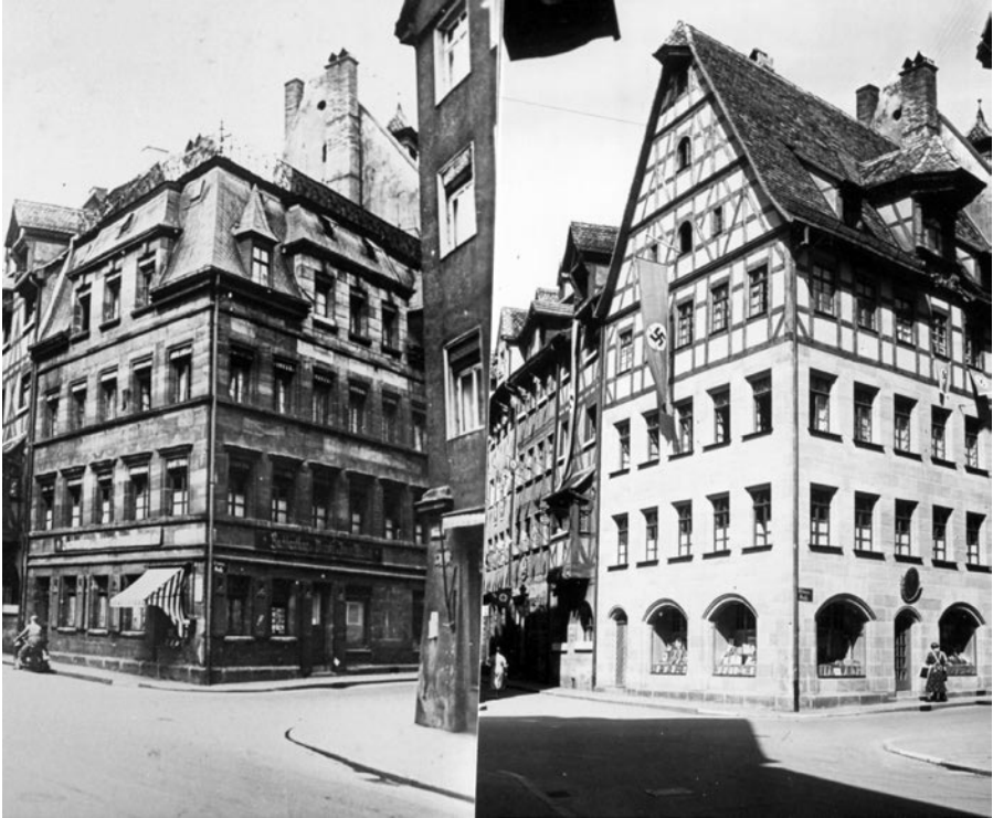
Figure 4.3. A Building in Downtown Nuremberg before and after Renovation
