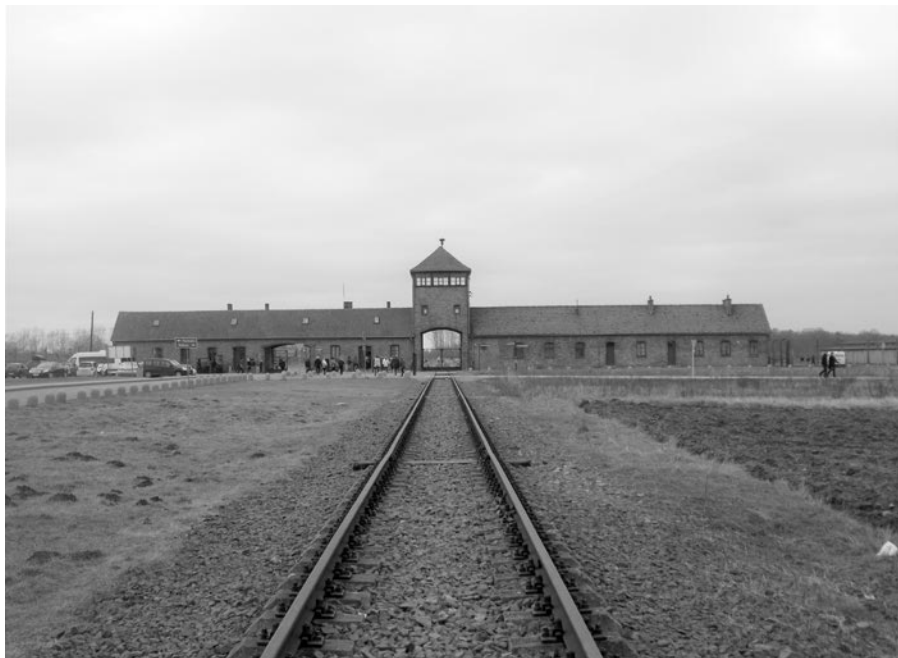
Figure 7.14. The Gatehouse Main Entrance to Birkenau
