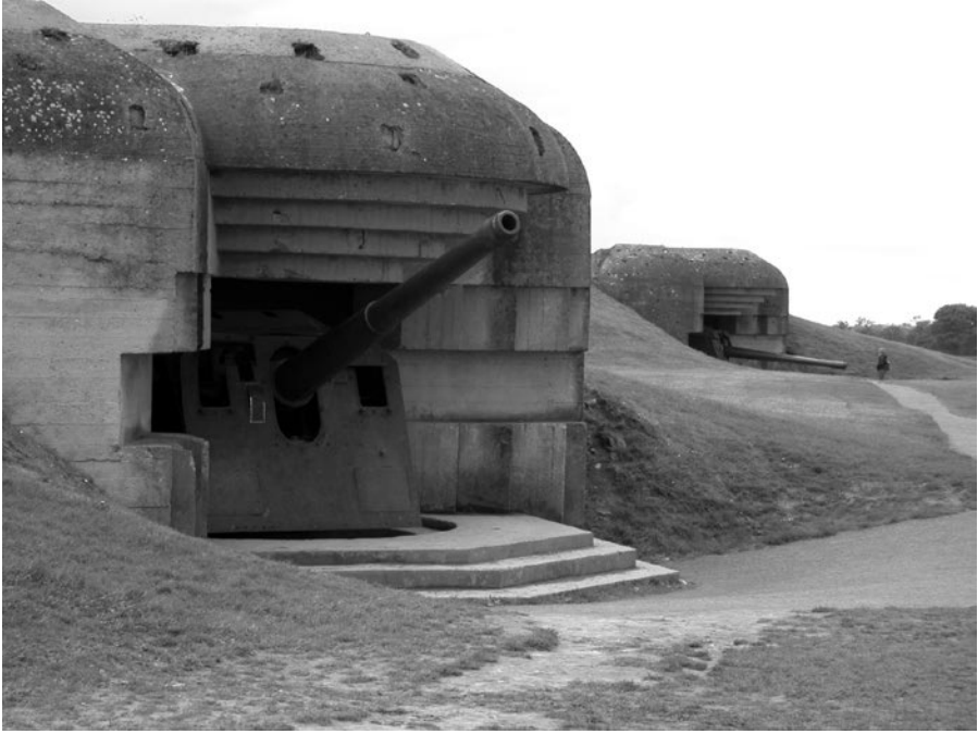
Figure 6.20. Massive Gun Emplacements as Part of the Atlantic Wall in Normandy
