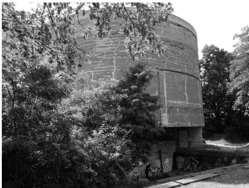
Figure 2.19. Massive Concrete Test Footing for Hitler's Planned Triumphal Arch
