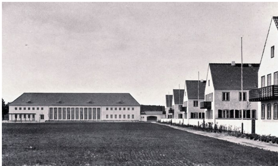
Figure 6.3. Worker Housing and Community Center at Heinkel's Oranienburg Complex
