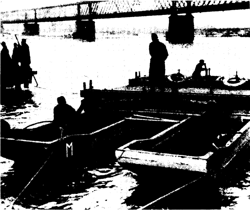
CONSTRUCTION of a German ponton bridge, 1941.
