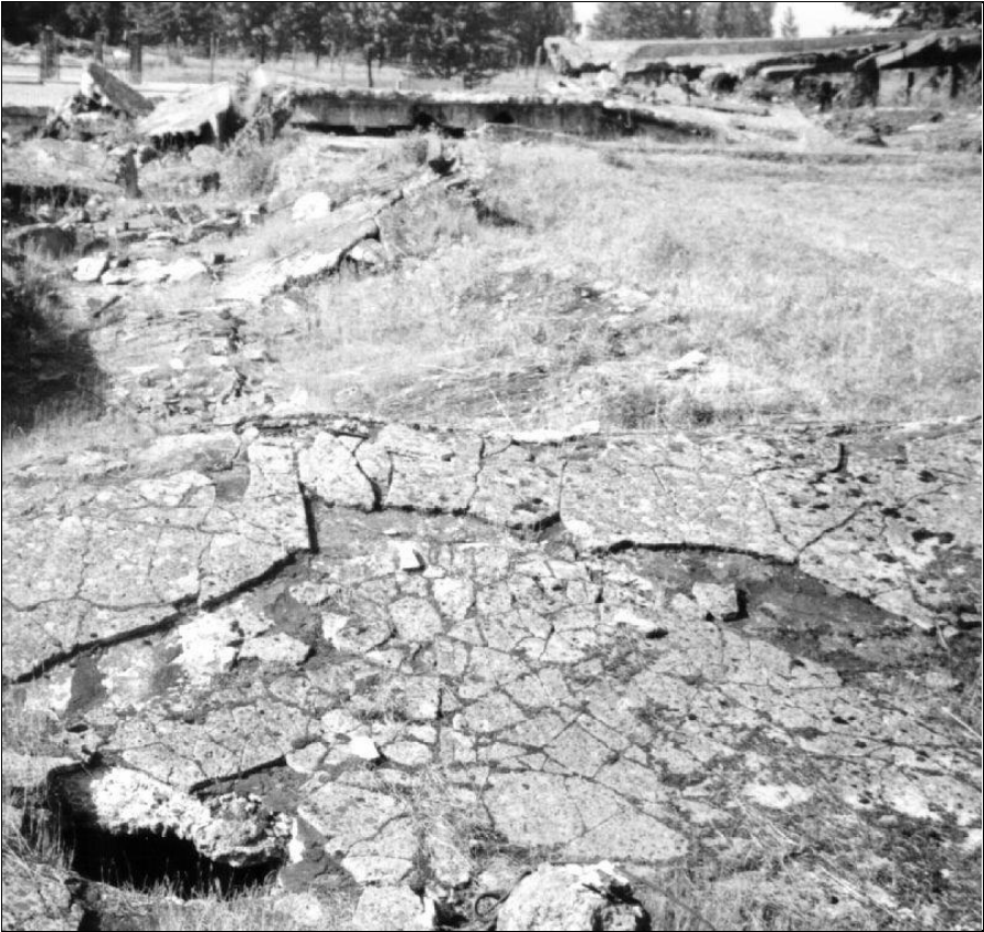
Illustration 15: The collapsed reinforced concrete roof of morgue #1 of Krema II at Birkenau in August 2000.
