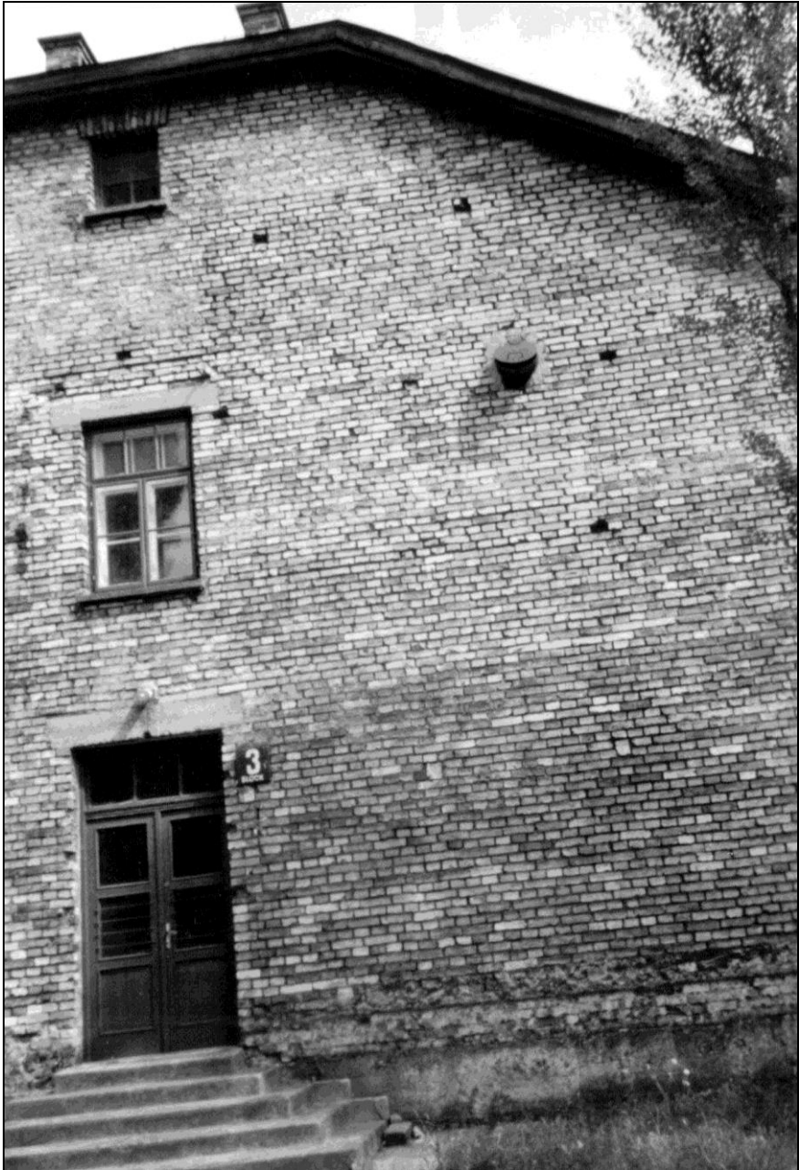
3. Auschwitz, Block 3. Round opening covered by a metal lid, which housed the ventilator for the gas disinfestation chamber located on the second floor of the Block. July 1992, © Carlo Mattogno.
