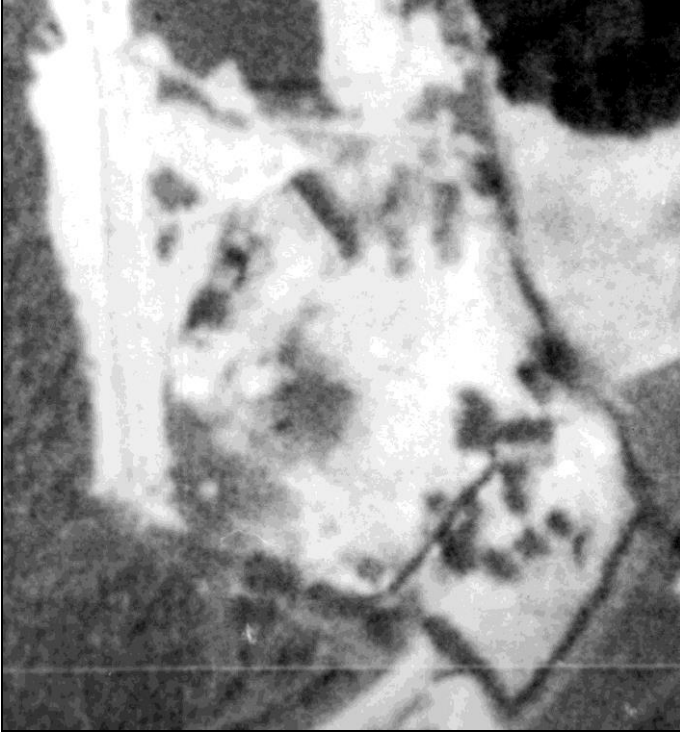
9b. Enlargement of photograph of May 31, 1944, pentagonal area of 'Bunker 2.'
