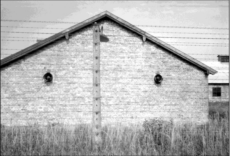
1. Birkenau, BW 5b, round openings for placement of ventilators in the outside wall of the gas disinfestation chamber. July 1992, © Carlo Mattogno.
