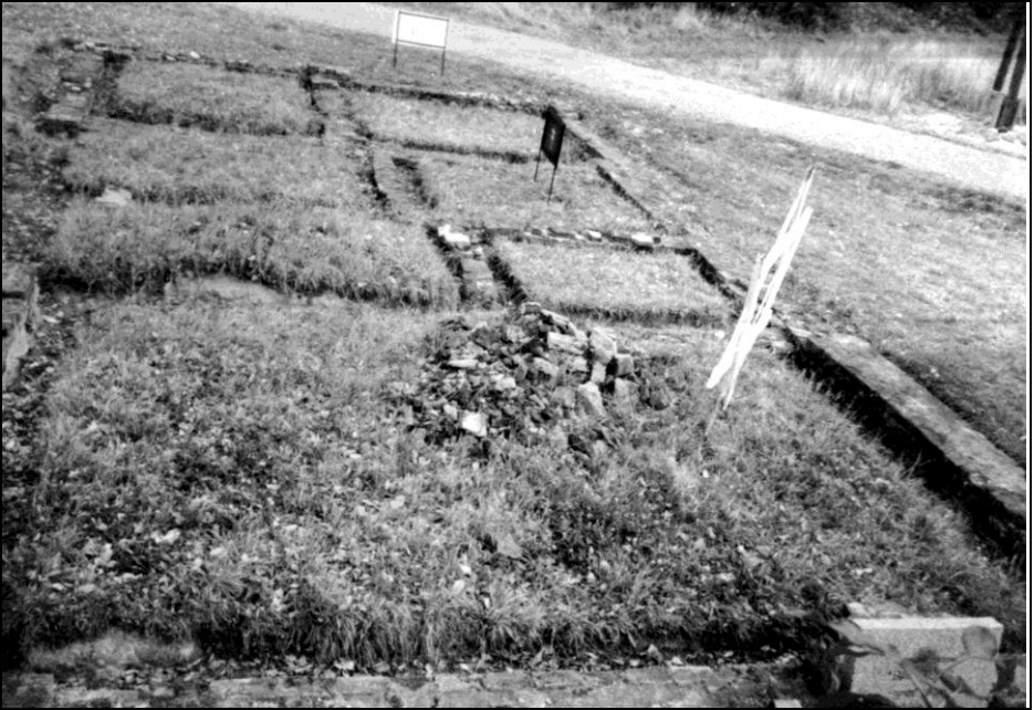
8. The ruins of the alleged 'Bunker 2' seen from the east. July 1992, © Carlo Mattogno.
