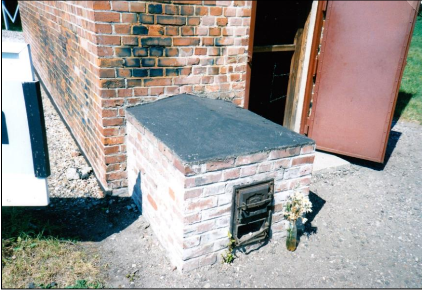
Photo 5: Delousing chamber at Stutthof, viewed from the south. The stove was used to heat the air inside the delousing chamber.
