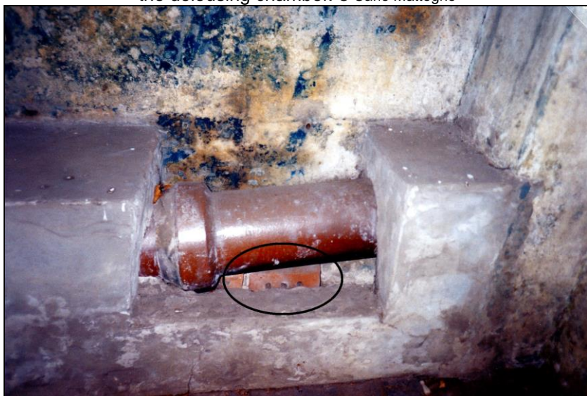
Photo 8: Delousing chamber at Stutthof, interior view, west wall; cast-iron connection pipe to the stove located outside the delousing chamber and used to heat the air inside the chamber. The pipe was originally surrounded by masonry similar to that visible in the photograph, but of perforated brick. One of these bricks is still visible today, underneath and behind the pipe (circle). © Carlo Mattogno
