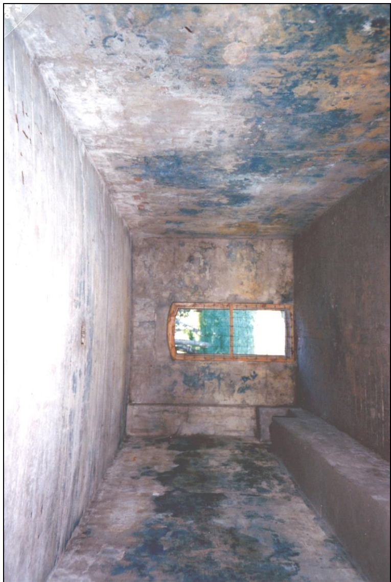
Photo 14: Delousing chamber at Stutthof, interior view from the south door. All the walls exhibit the typical blue pigmentation caused by iron cyanide. © Carlo Mattogno
