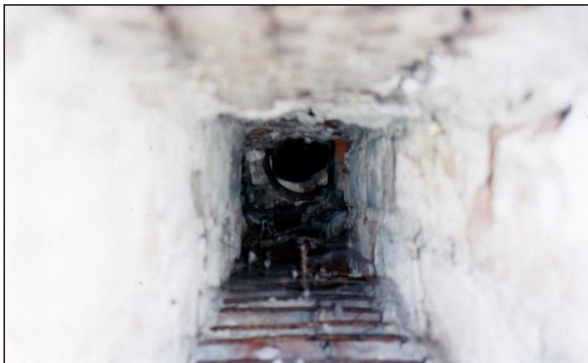
Photo 7: Delousing chamber at Stutthof, viewed from the south. The stove was used to heat the air inside the delousing chamber. Interior view of the combustion chamber. Beneath: the plane grid; above: the circular opening of the connection to the cast-iron pipe located inside the delousing chamber. © Carlo Mattogno
